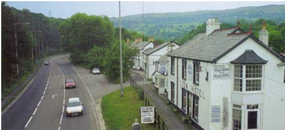
Lion Hotel and Terrace at Gilwern would be demolished
