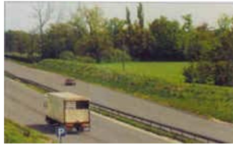
Mounding and planting on recently constructed road
