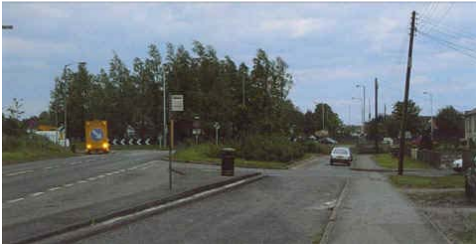
Road works at Hirwaun
