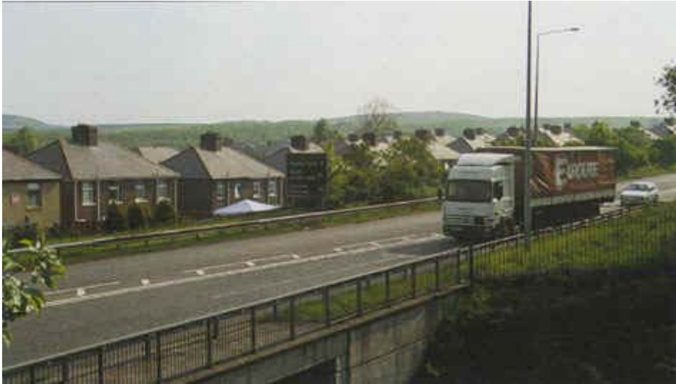
Housing close to existing route at Rassau
