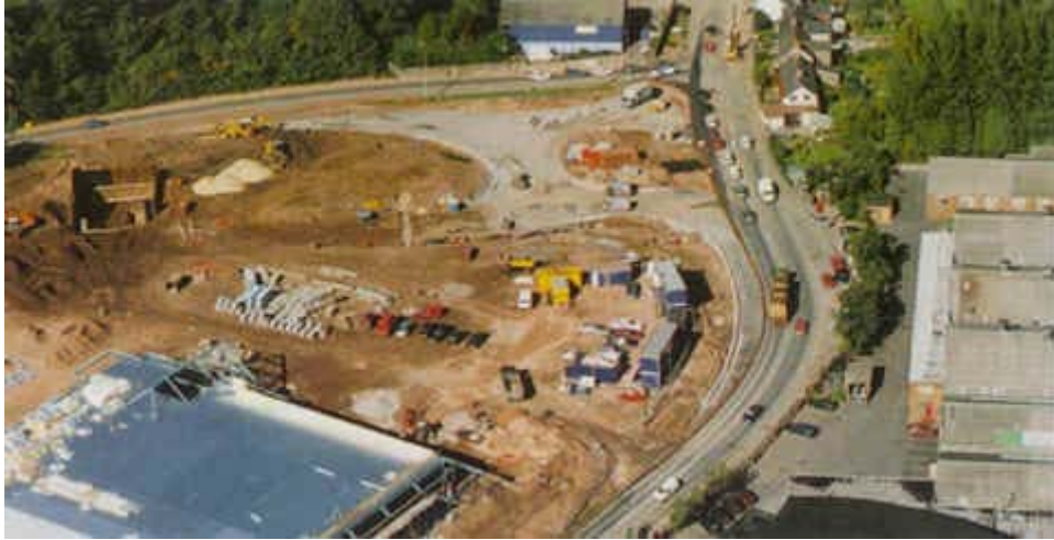
Construction in progress at Llanfoist
