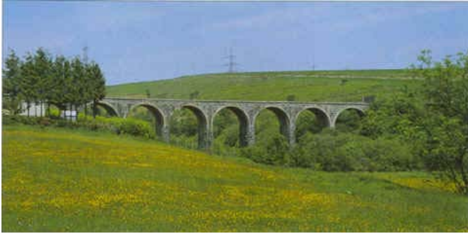
Railway Viaduct near Nant-y-Bwch
