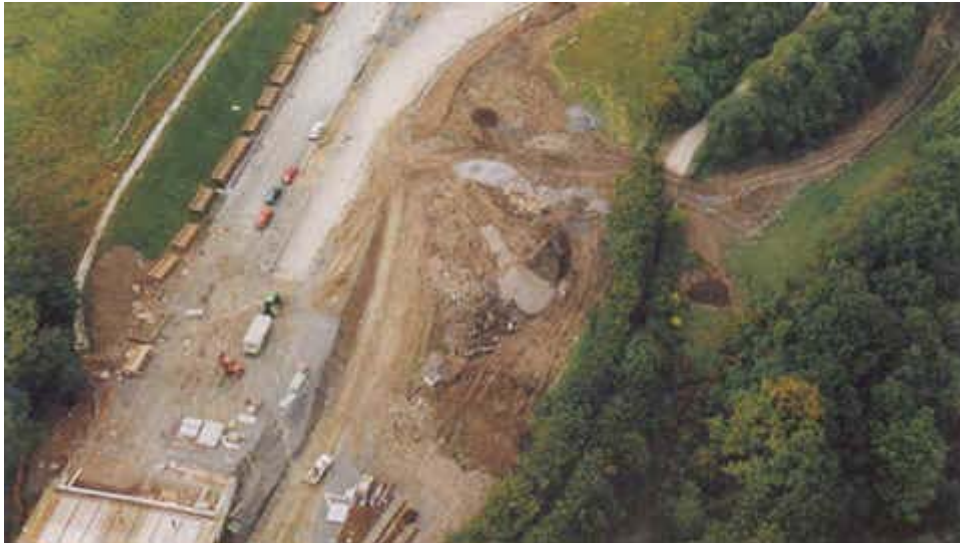
Construction of new A470 at Cefn Coed-y-Cwmmer
