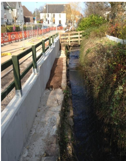
Figure 4: Flood alleviation works, Rhiwbina, Cardiff
