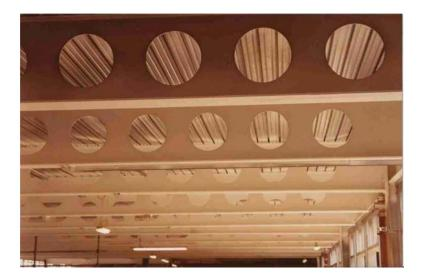
4.5 Photograph 2 shows the beams and profiled steel sheets on an unaffected part of the building.
