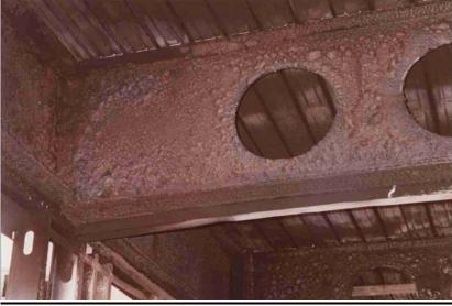
4.7 Photographs 4 & 5 show the beams immediately above the fire area on the ground floor.
