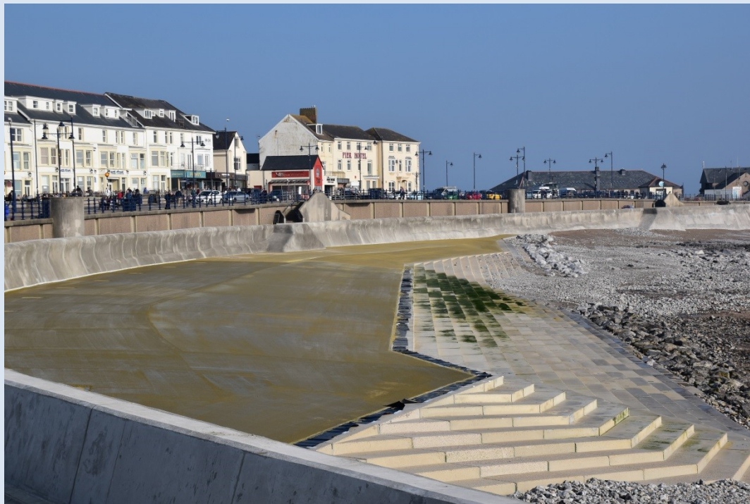
Porthcawl Town beach coastal scheme, completed in 2019.
