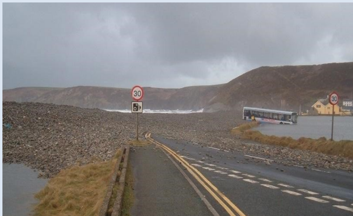
Damage at Newgale, Pembrokeshire blocking coastal road
