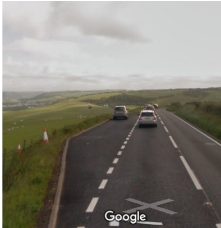
A487 Northbound layby
