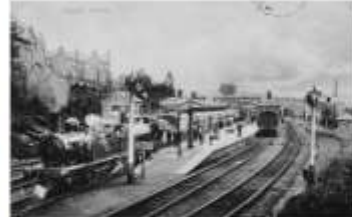
Original "Refresh" in the far distance, also original footbridge which we plan to reinstate. This also shows the Island Platform being used much as we propose.
