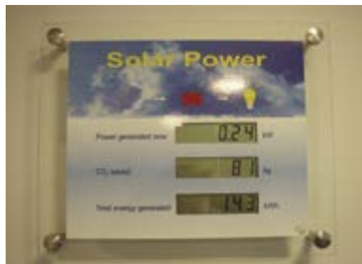
Photovoltaic output display at Canolfan Hyddgen © Reproduced with permission of Powys County Council
