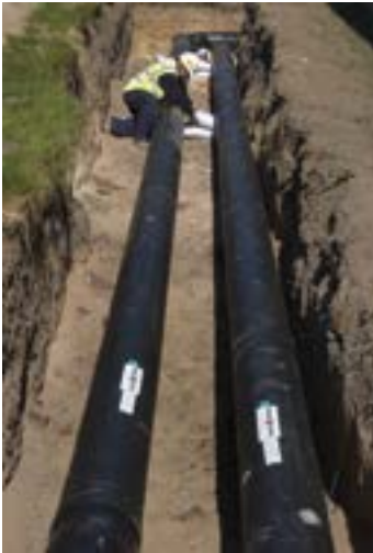
Installation of distribution pipes Reproduced with permission of Aberdeen City Council
