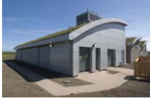
CHP Energy centre at Seaton Reproduced with permission of Aberdeen City Council
