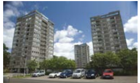
Multi storey apartment blocks in Aberdeen Reproduced with permission of Aberdeen City Council
