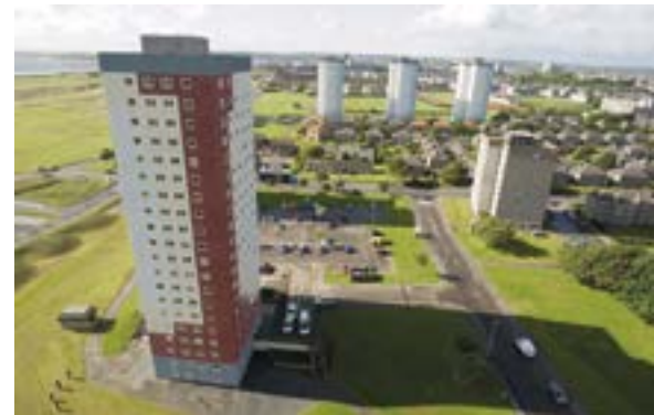
Multi-storey housing developments linked to the district heating scheme. Reproduced with permission of Aberdeen City Council
