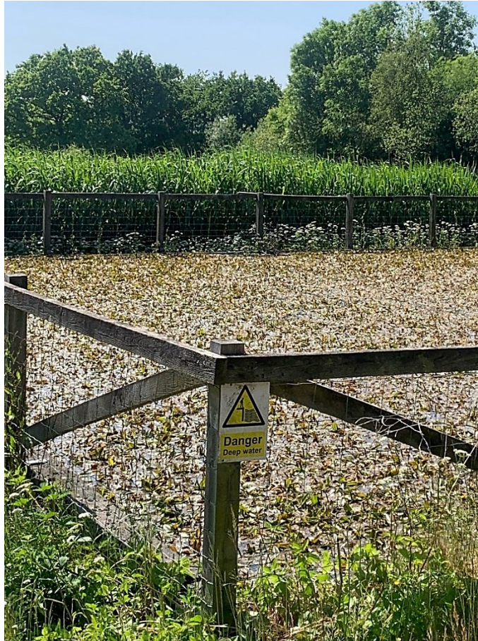
Coed Top reed bed water treatment facility.
