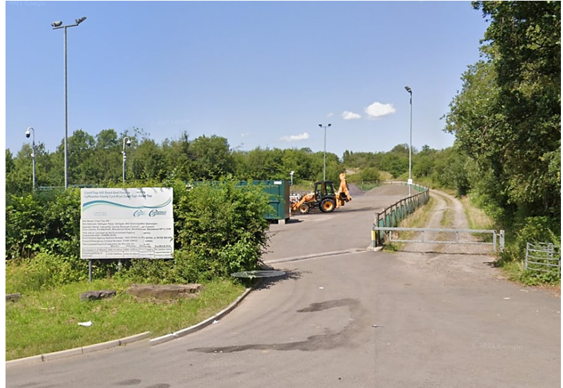
'Caerogen' Project site entrance.
