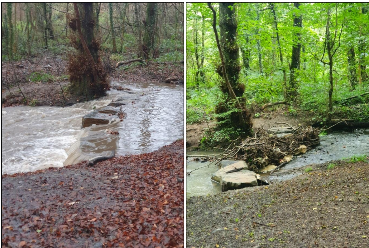
Figure 4 Site 1 Preswylfa Dingle stepping stones capturing debris in high flow.
