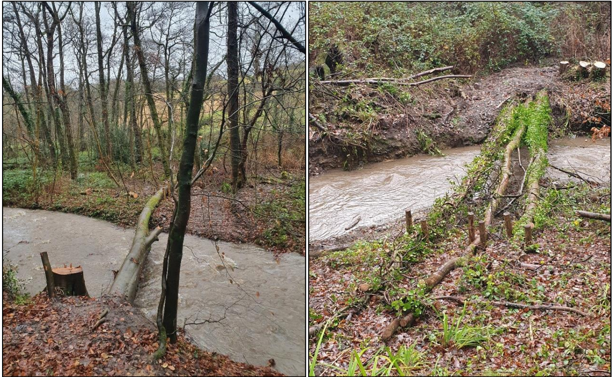
Figure 3 Site 1 Preswylfa Dingle post leaky barriers implementation and post flood event.
