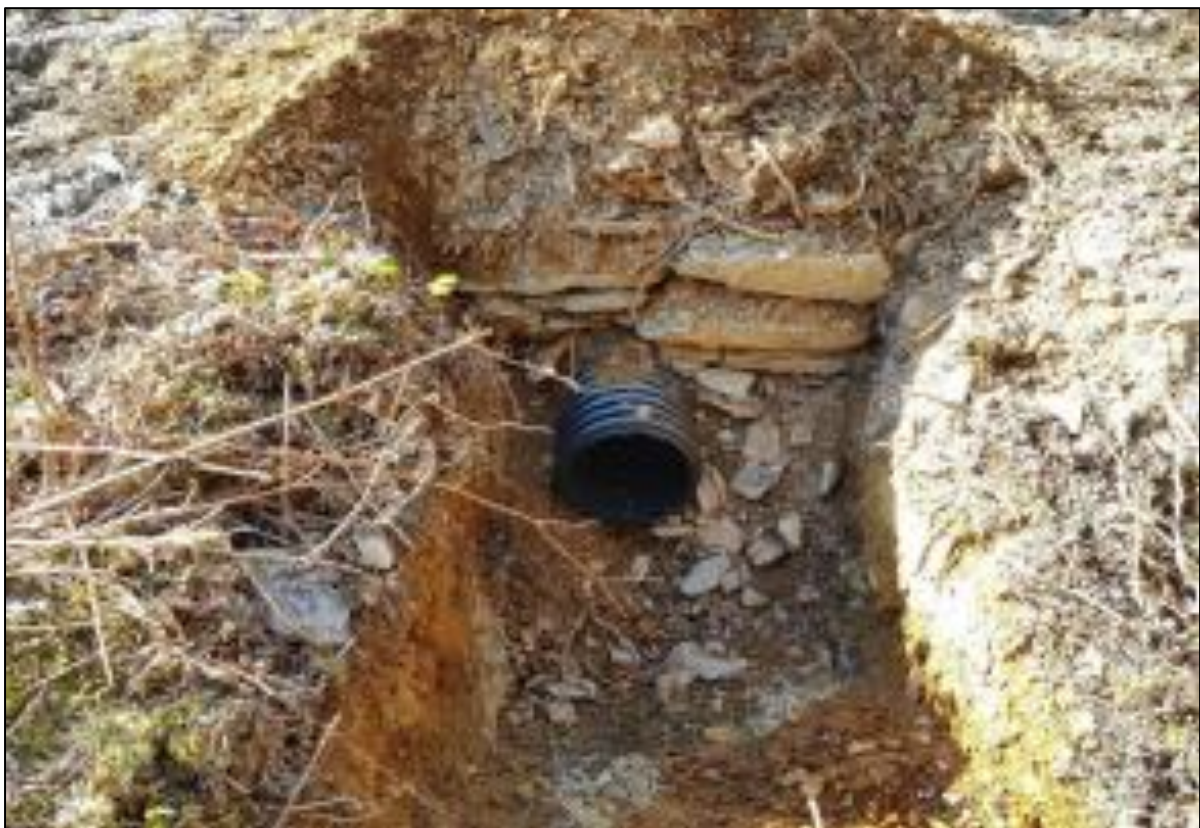
Figure 4 Example of a new flow control culvert implemented as part of the scheme.
