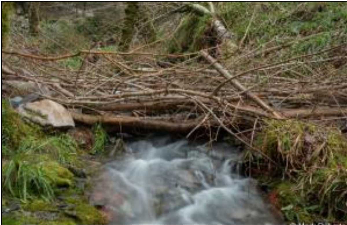
Figure 3 Example of a leaky barrier implemented as part of the project.
