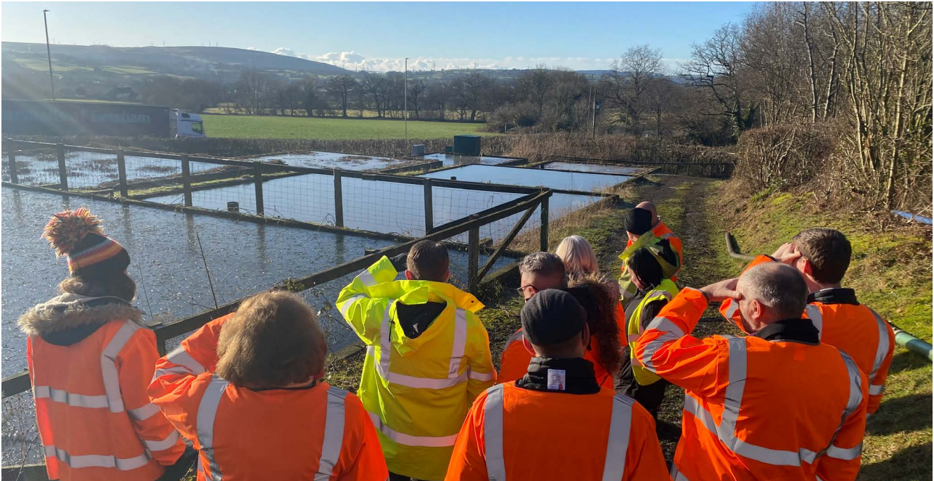
Reed bed settling tanks at the Coed Top Caerogen trial site.
