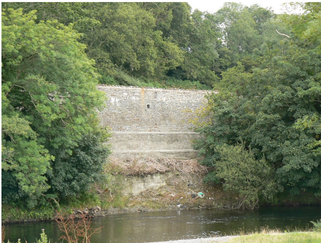
Photograph 15 – Retaining structure supporting the existing A487
