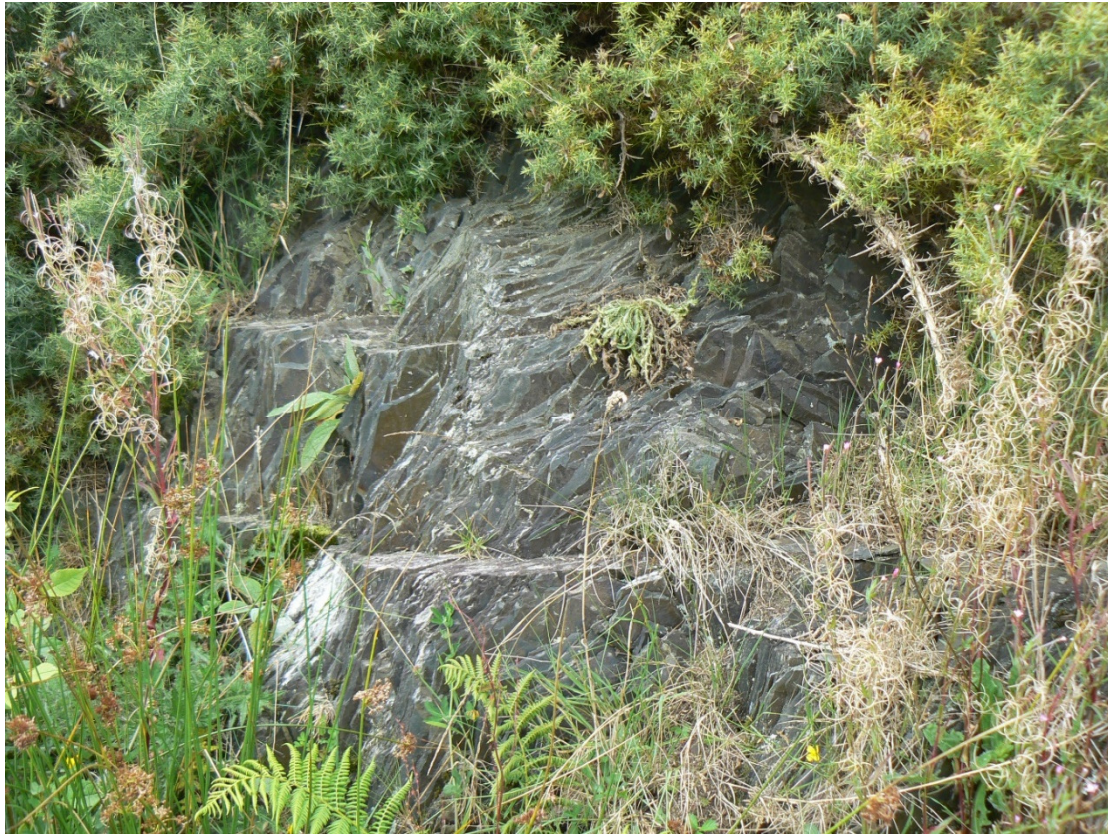
Photograph 18 – Vertical discontinuities in the rock cutting at around Ch. 1+100m
