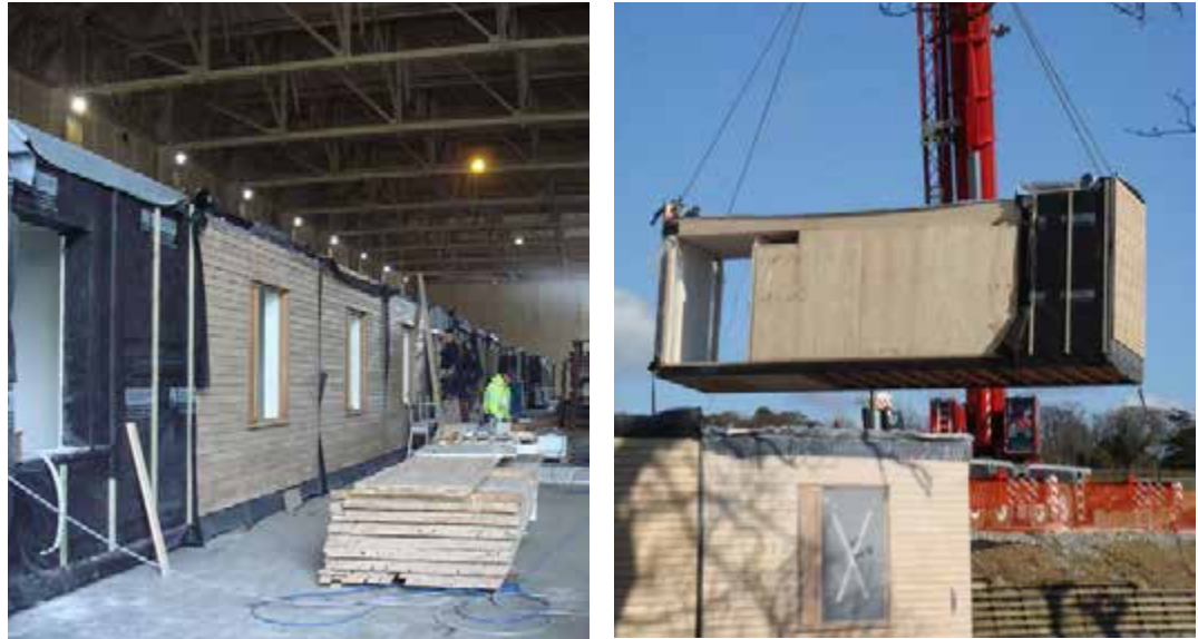
Fig 14: Factory-made module being lifted into place Images courtesy of DRU-W
