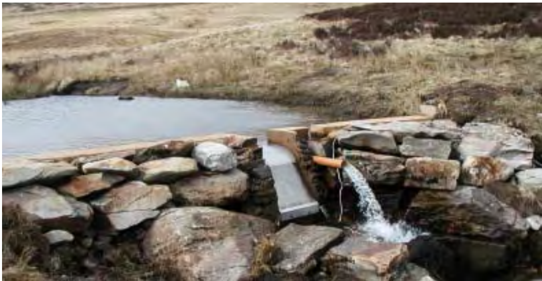
Figure 12: Intake weir on small run-of-river hydro scheme
