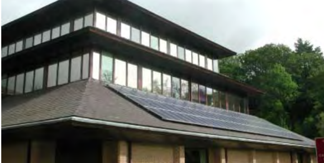
Figure 8: PV array retro-fitted to office complex
