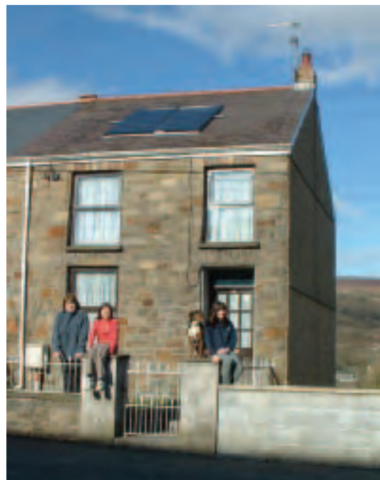
Figure 10: Flat-plate solar collectors
