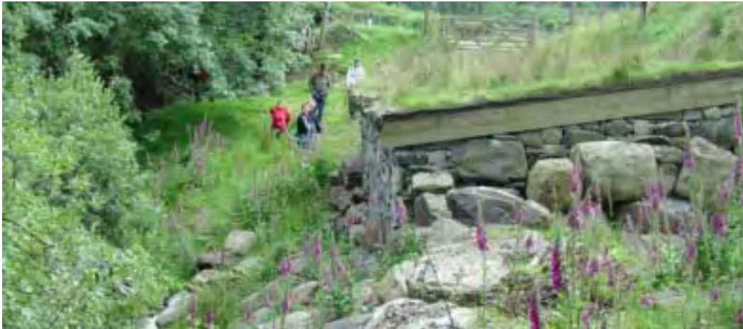
Figure 13: Turbine house on hydro scheme at Figure 12
