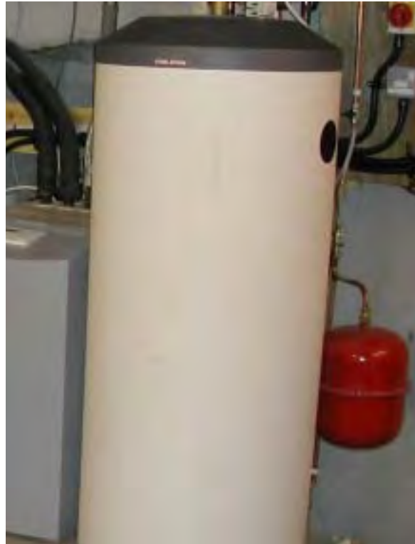
Figure 14: Domestic heat pump arrangement with buffer tank
