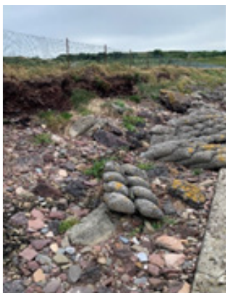
Prior to removal, these concrete pillows were unsightly debris that were inhibiting natural shoreline processes at this location
