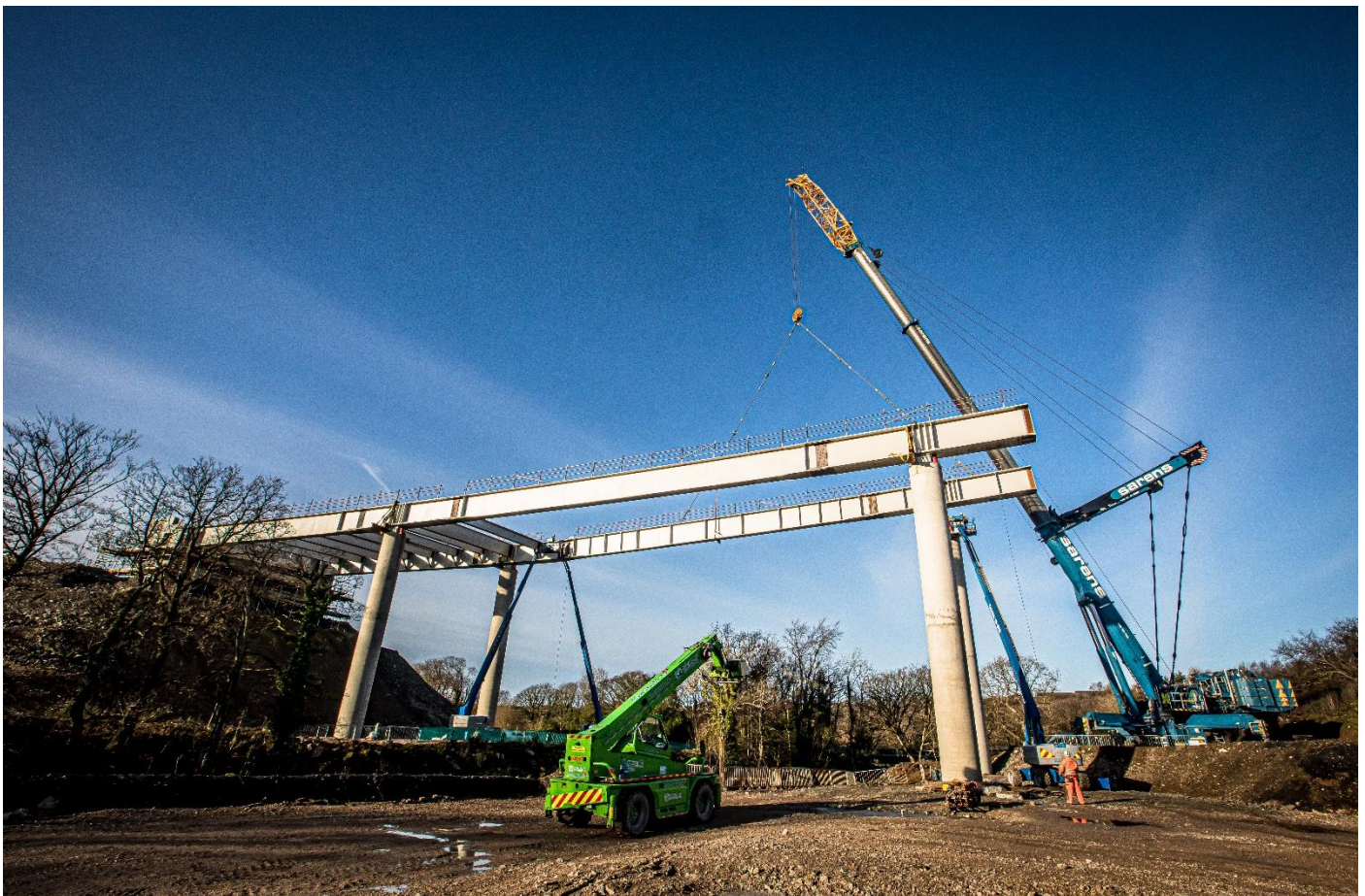
The viaduct crossing the River Seiont during construction, a 2m deep beam being lifted into position using a 750t mobile crane.
