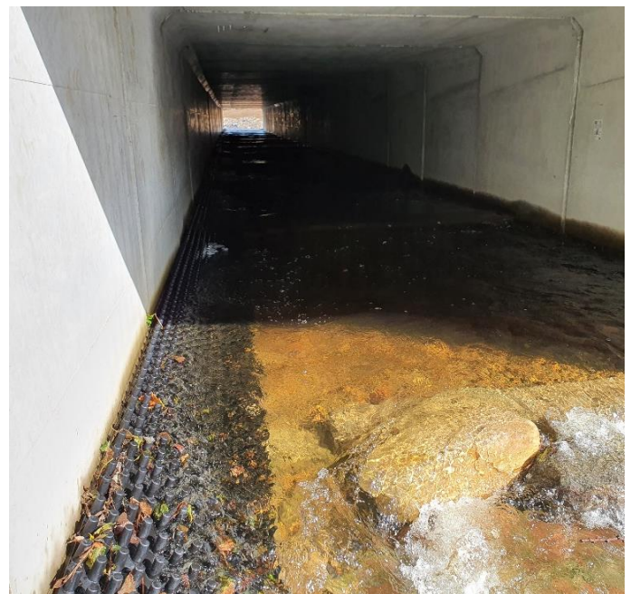
Afon Rhyd culvert includes fish baffles and elver matting to allow upstream passage of migrating fish and eels.
