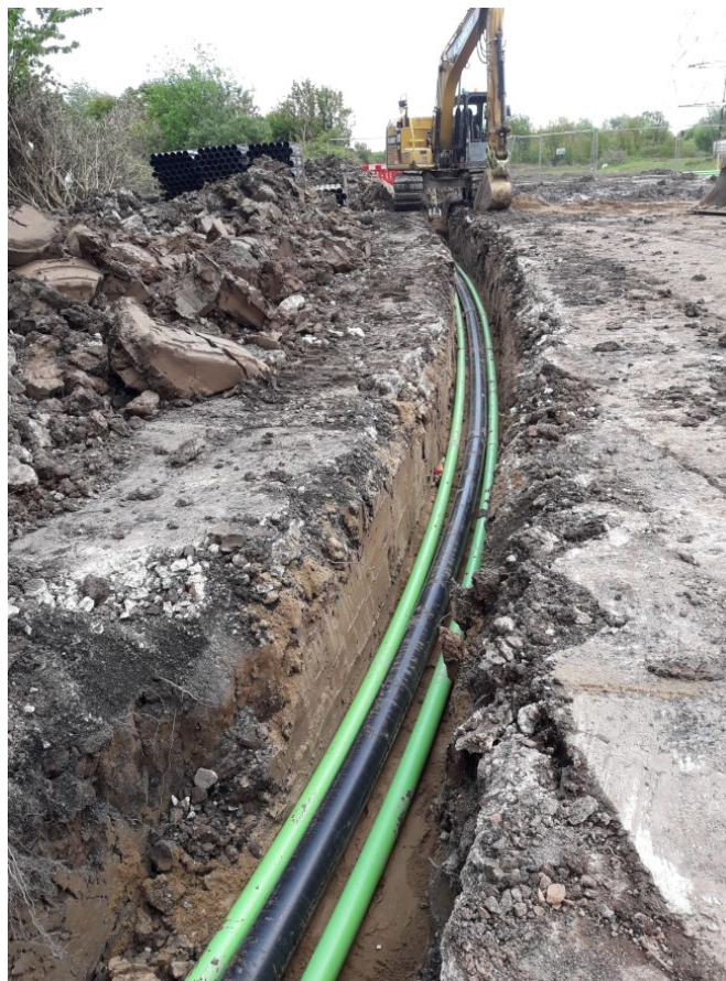
Figure 2 - Ducts installed at Launch Drill Location, Lamby Way, Cardiff City Council
