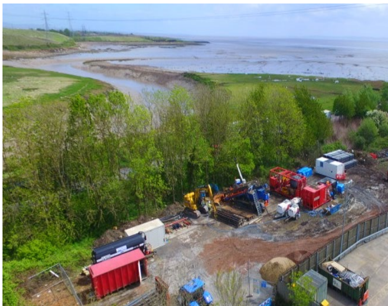
Figure 3 - Directional Drilling Plant – entry site on the River Rhymney estuary connecting Lamby Way solar farm to Welsh Water
