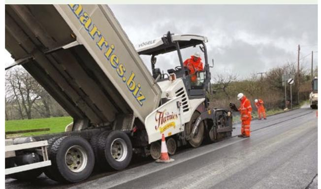
As part of Wales’ bid to become a zero waste nation by 2050, fibres from 4.3 tonnes of dirty nappies have been used in trials to resurface a stretch of road on the A487 between Cardigan and Aberystwyth.
