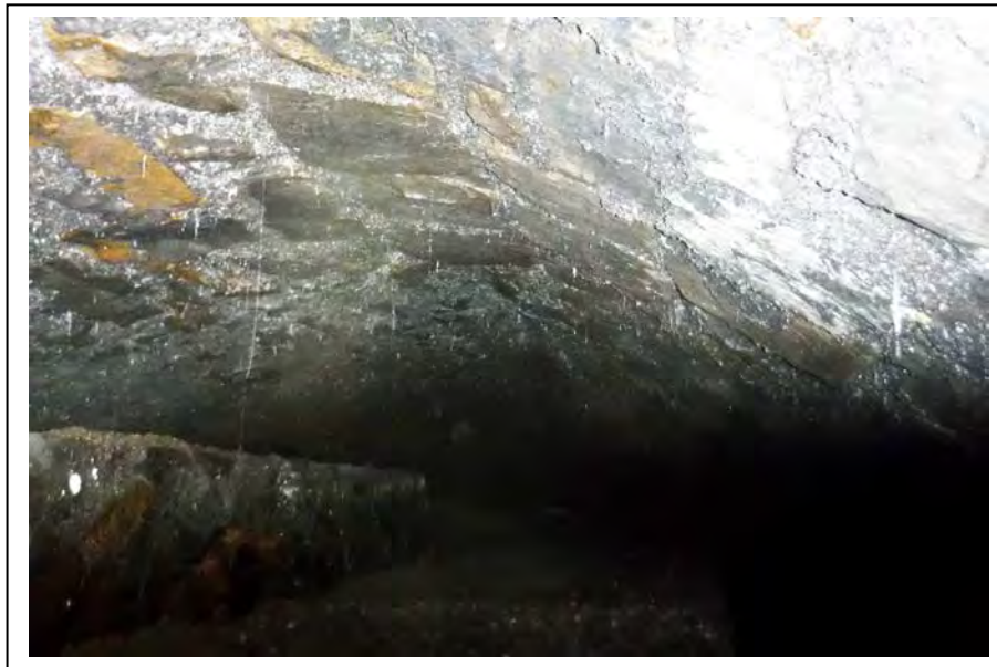
Photograph no C48: Form of barrel only slightly hinged at CE of Cwg ③
