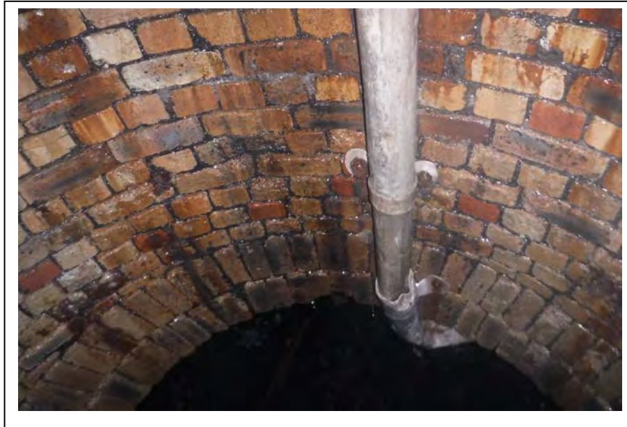
Photograph no 181: Remaining down-pipe to lower section of shaft
