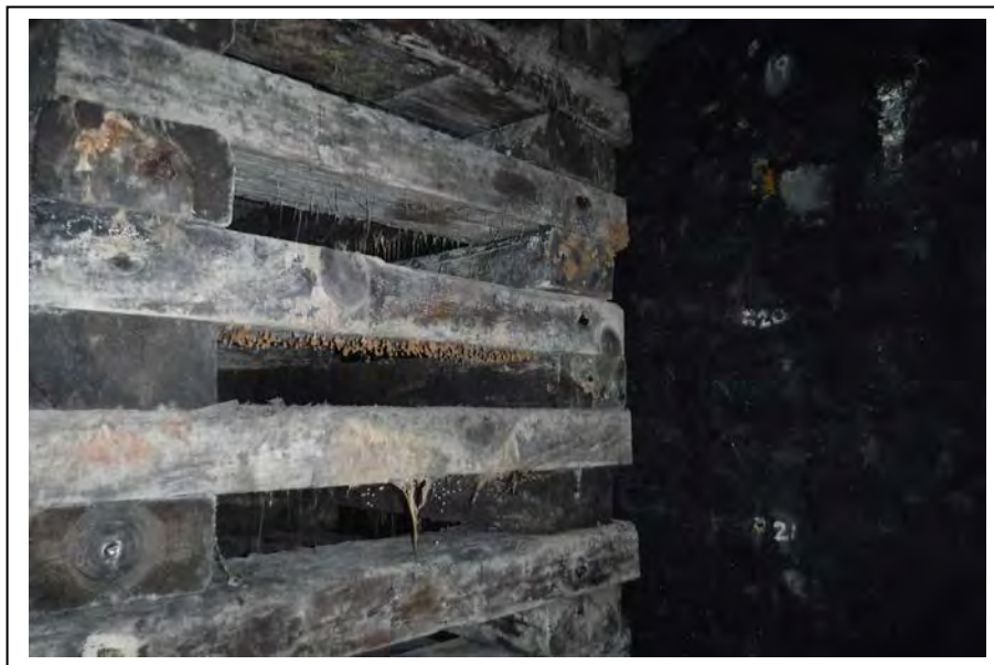
Photograph no C12: Cwg ② CE sidewall
