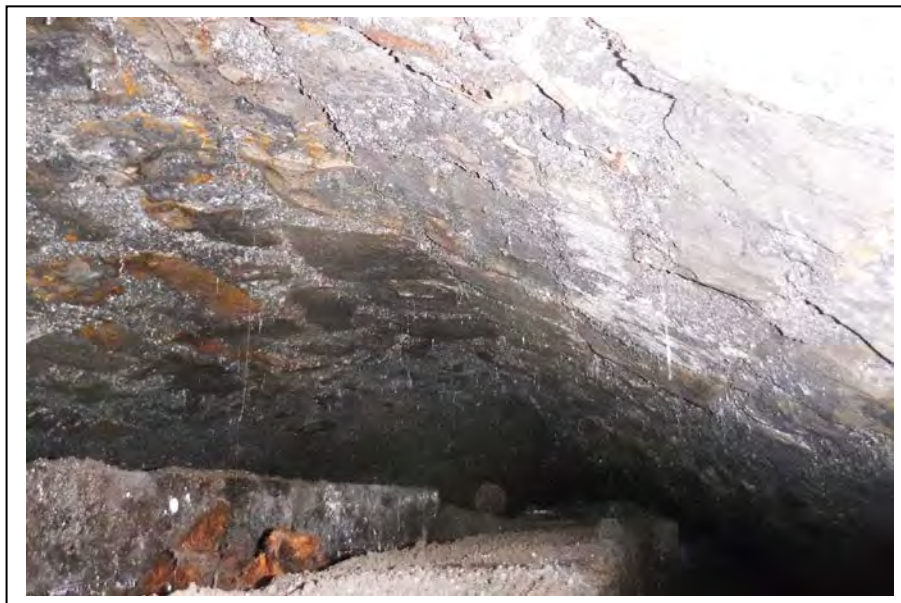
Photograph no C46: Form of barrel only slightly hinged at CE of Cwg ③
