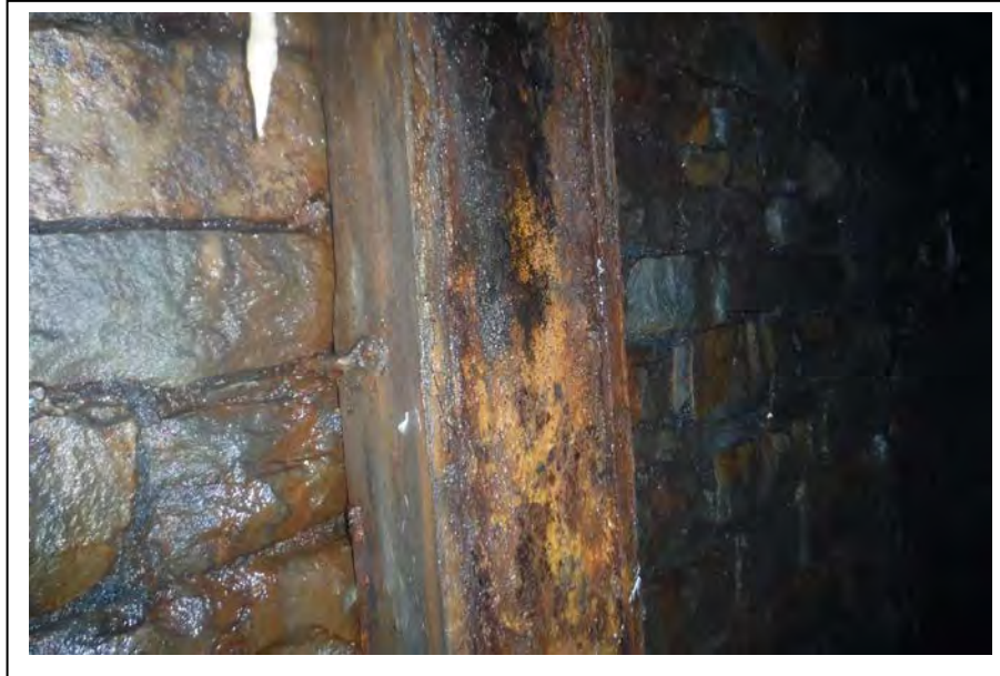
Photograph no 189: Down-pipe appears functioning
