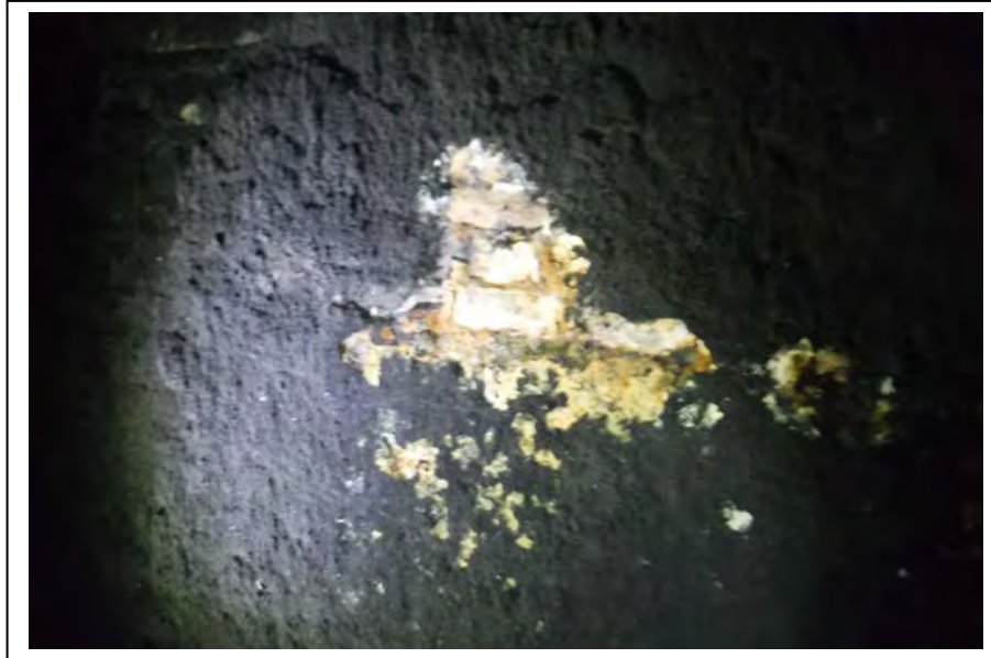
Photograph no 145: D/S sidewall at 2475m Soft concrete repair to surface
