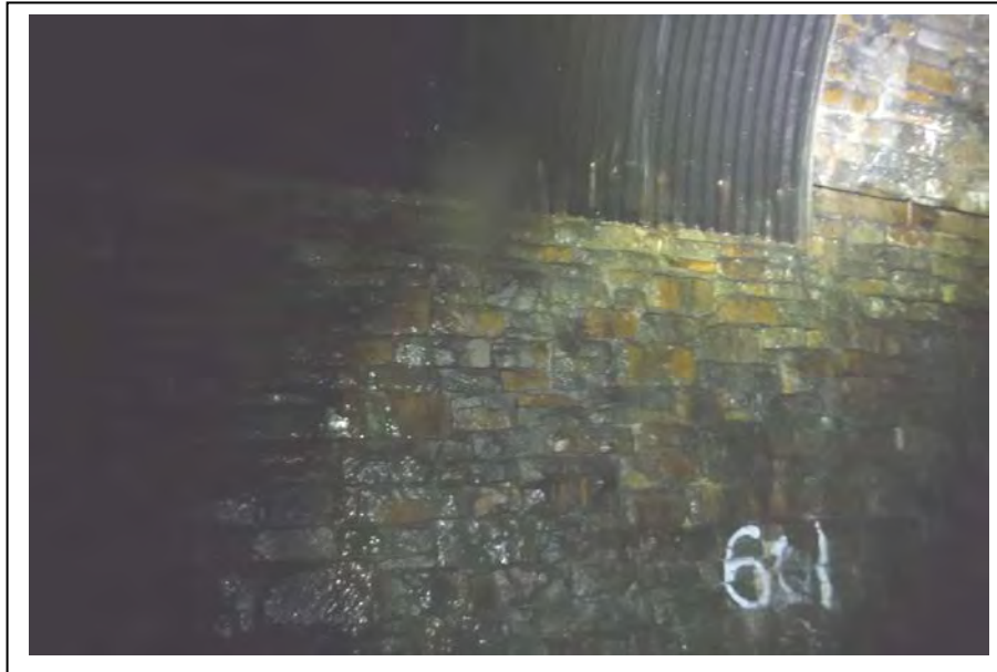
Photograph no 13: Corrugated metal sheeting at 64m
