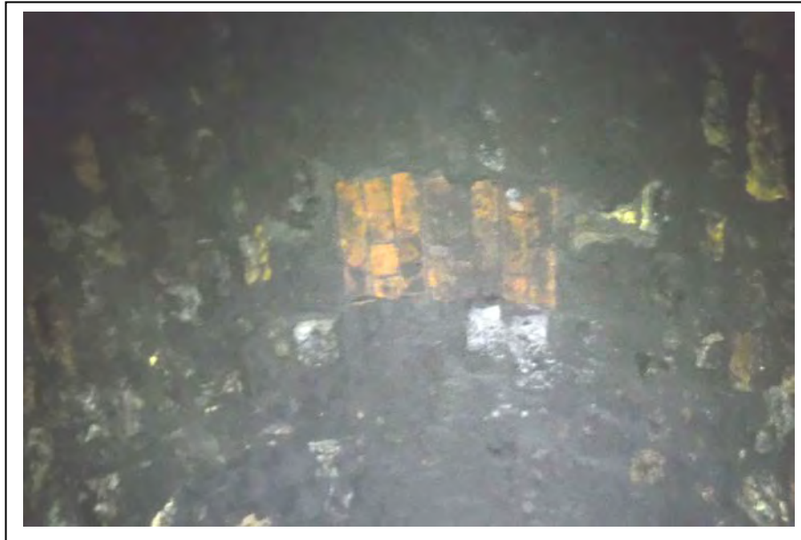
Photograph no 55: Crown at 290m Brick repair firm to hammer
