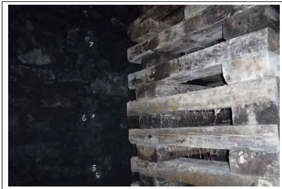
Photograph no C13: Cwg ② CE sidewall
