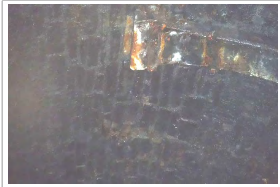
Photograph no 187: Crown at 3052m Metal drainage hopper and down-pipe
