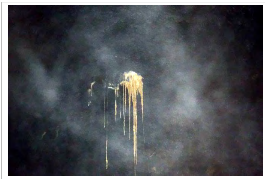
Photograph no 200: Crown at 3082m Stalactites
