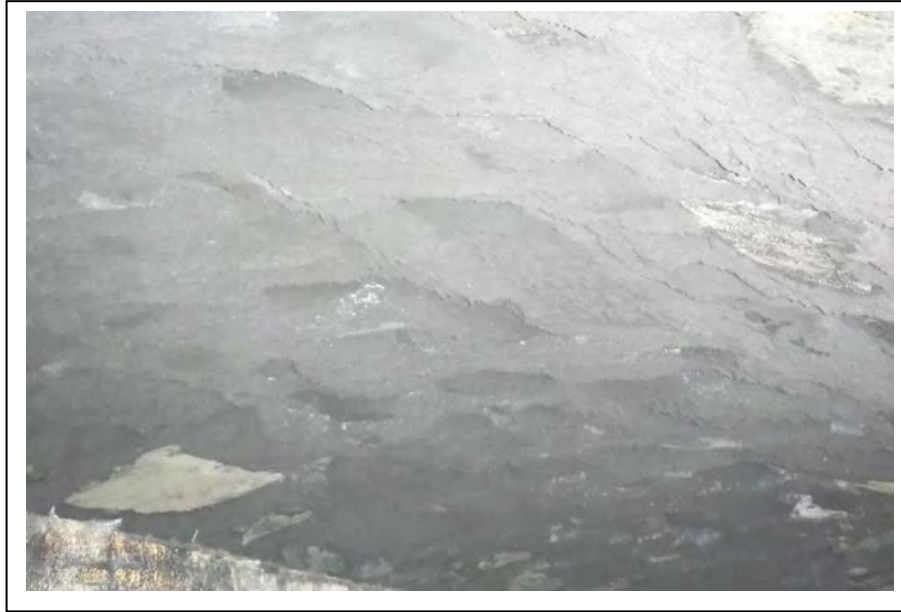
Photograph no C21: Hinge to crown visible at LE
