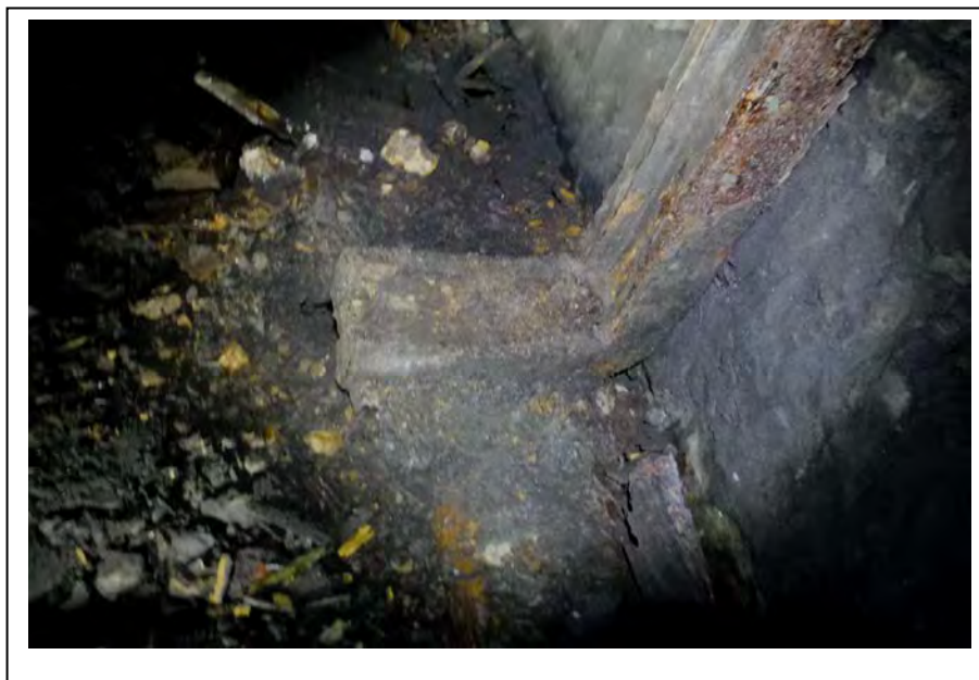
Photograph no 76: Cranked rib showing connection at base
