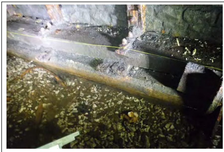
Photograph no 72: Bulk timbers to base of rib support
