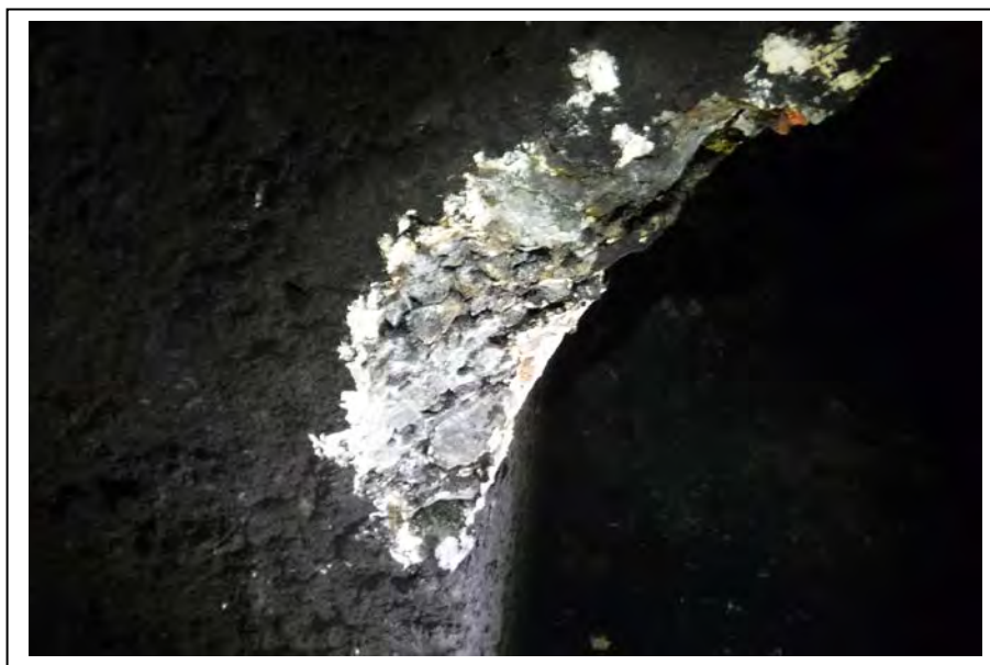
Photograph no 122: U/S refuge at 1160m Spalling 140 deep x 120 wide x 500 long to relieving arch
