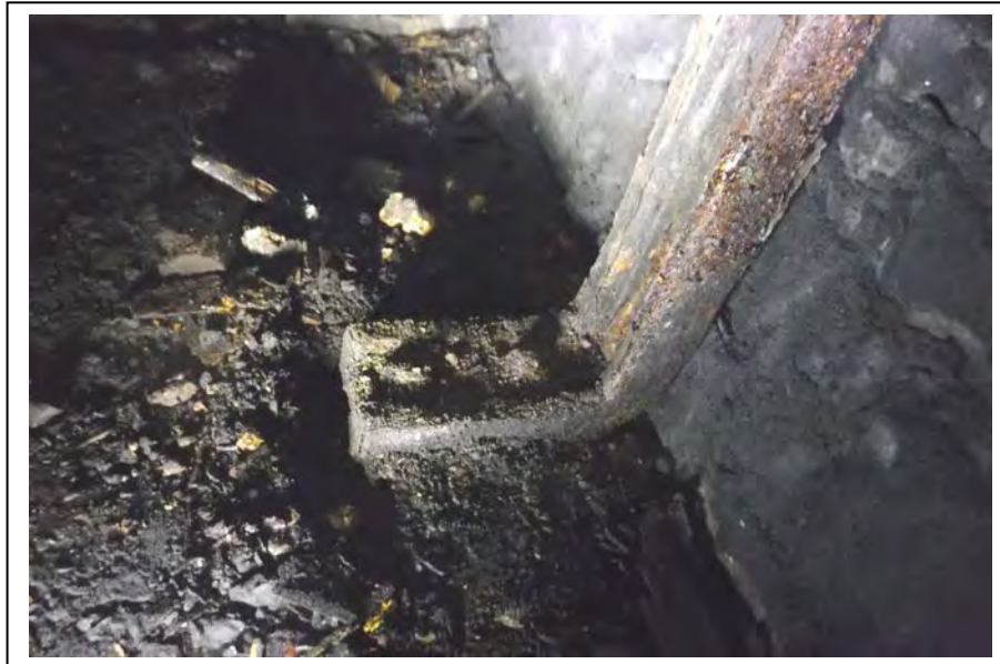
Photograph no 77: Cranked rib showing connection at base
