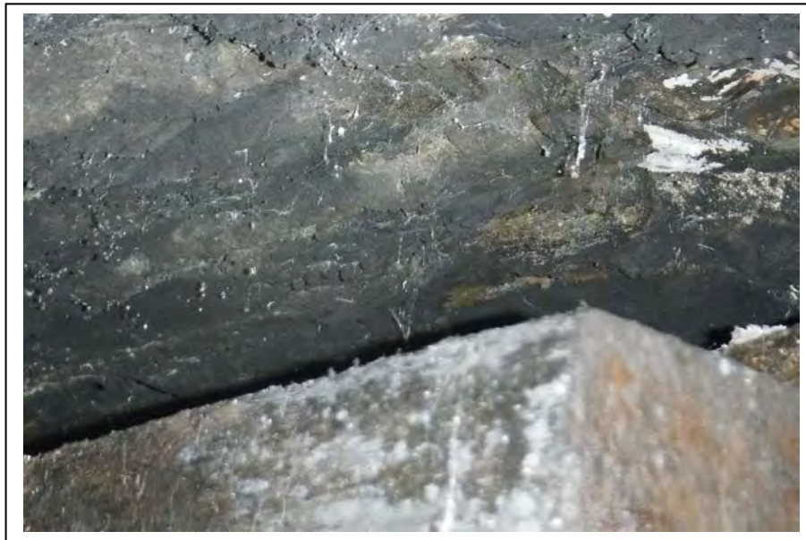
Photograph no C32: No evidence of packing to haunches of Cwg gap is typical of all elements, similar to crown
