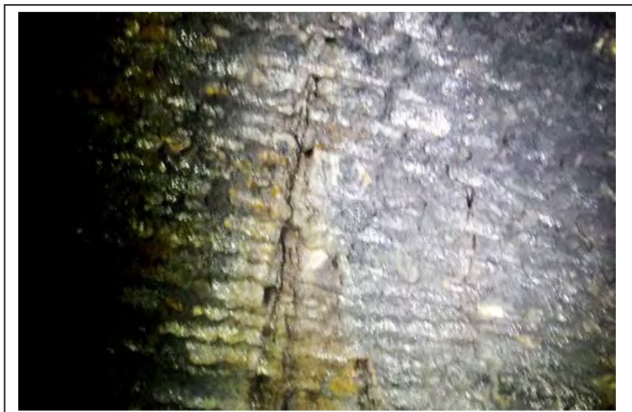
Photograph no 152: Crown at 2980m Construction joint
