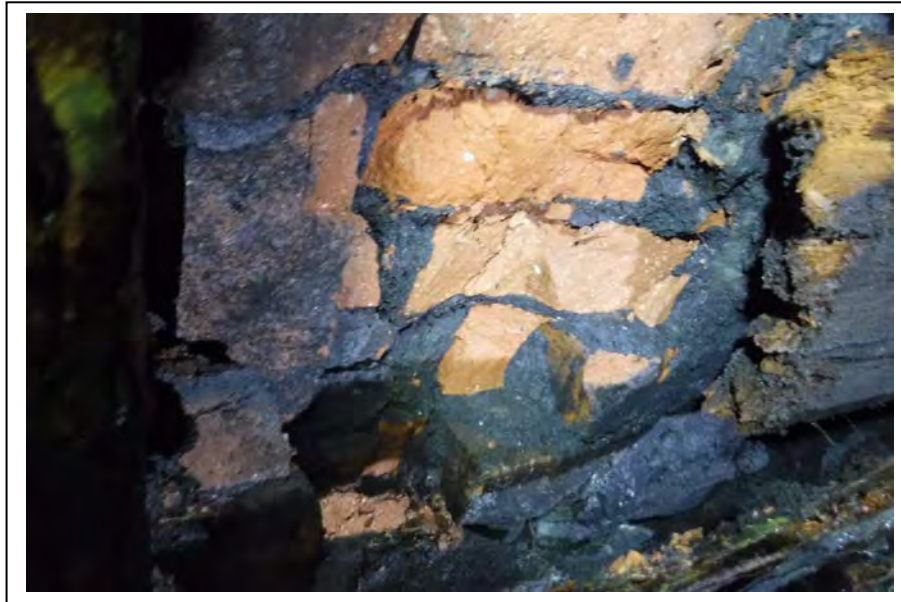
Photograph no 103:U/S crown at 981m – 983m (Ribs 44-46) Loss of section 1m 2 x 180 deep max
