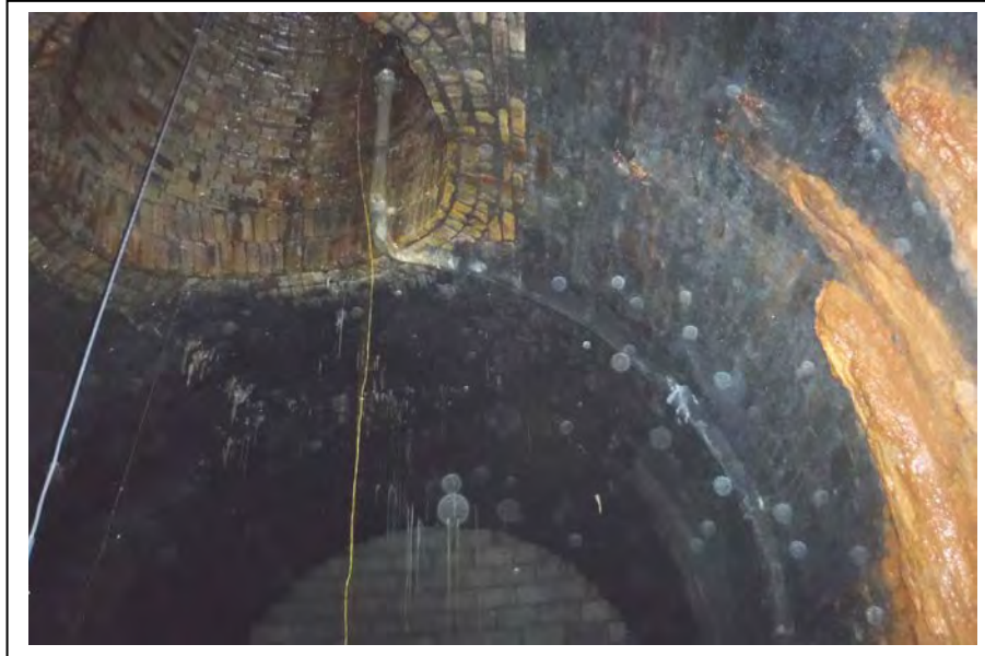
Photograph no 161: D/S sidewall to crown at 3037m Drain-pipe to shaft
