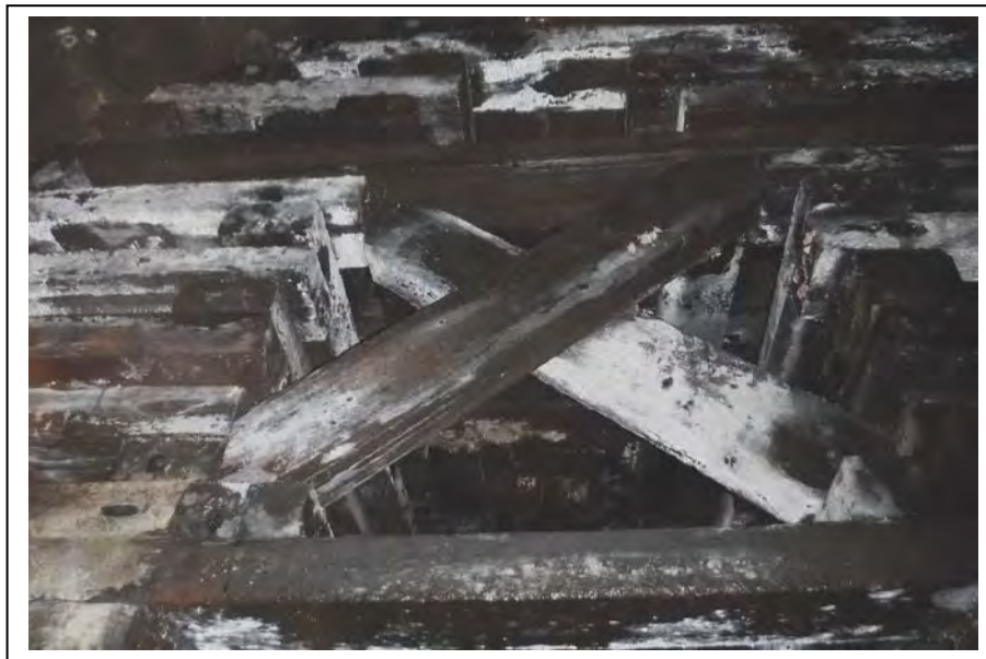
Photograph no C11: Cwg ② CE crown
