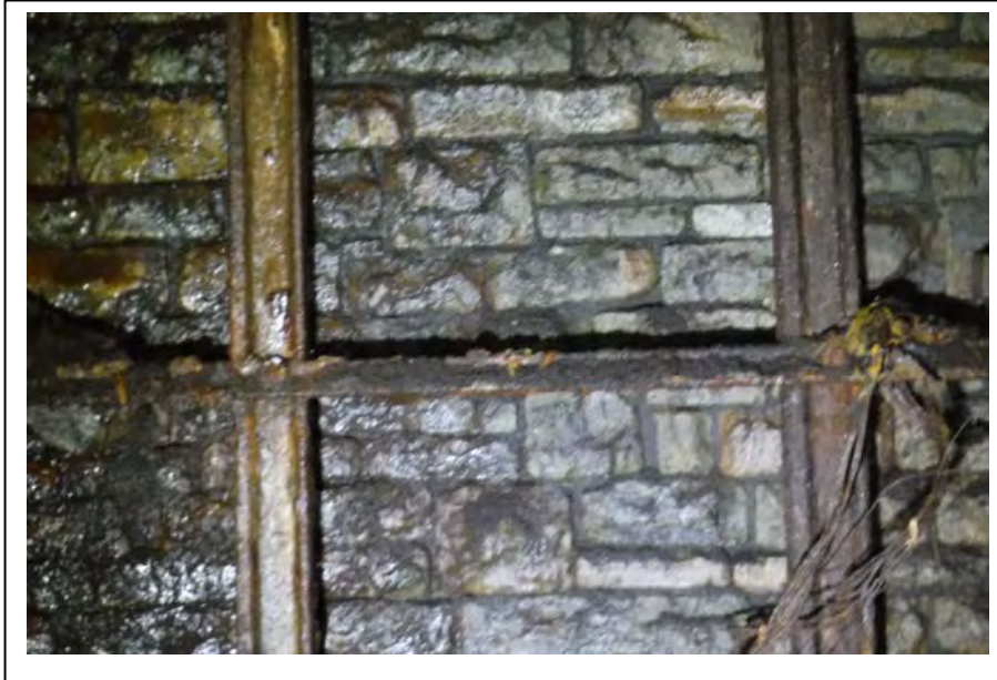
Photograph no 69: Typical view of ribs and horizontal bracing
