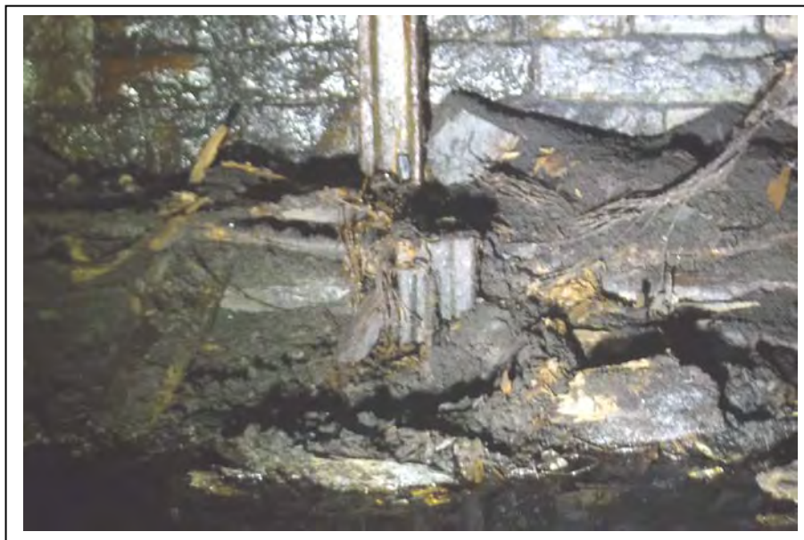
Photograph no 68: Typical rib and vertical pile support (below ground)
