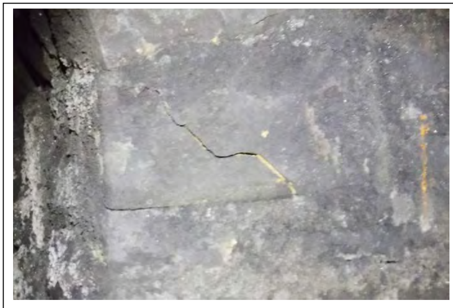
Photograph no 108: Refuge at 1020m Single fractured unit to D/S quoin open to 3mm
