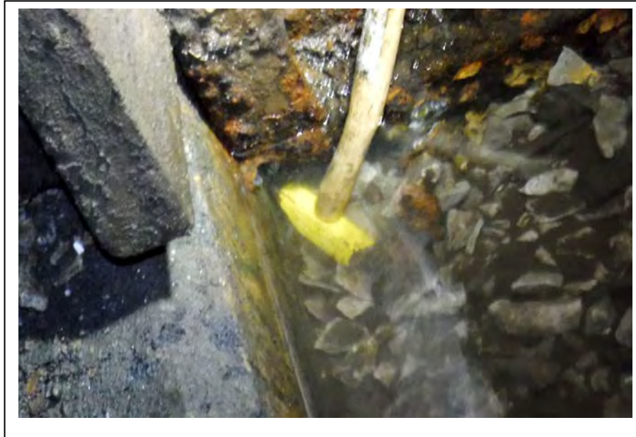
Photograph no 71: Base of strut and column support (typical)
