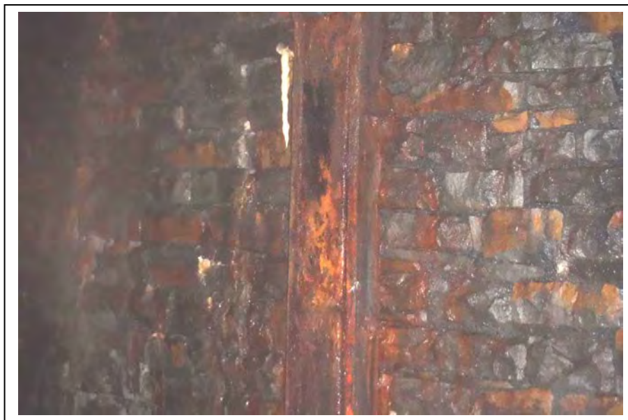
Photograph no 188: U/S sidewall to crown at 3052m Down-pipe
