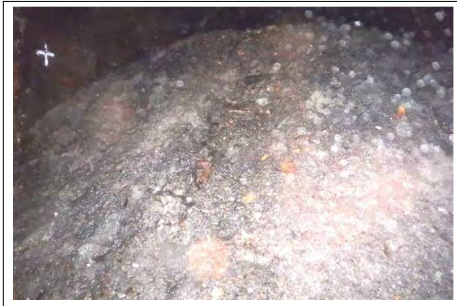
Photograph no 207: Tunnel back-filled to haunch level Sidewalls not examined after 3010m
