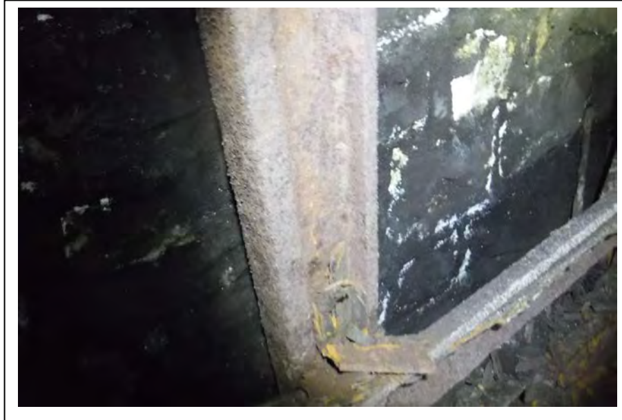
Photograph no 67: Typical rib section
