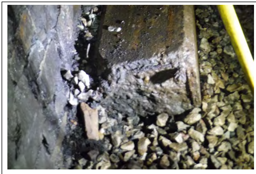
Photograph no 52: D/S sidewall at 210 – 225m Redundant concrete beam at base of sidewall
