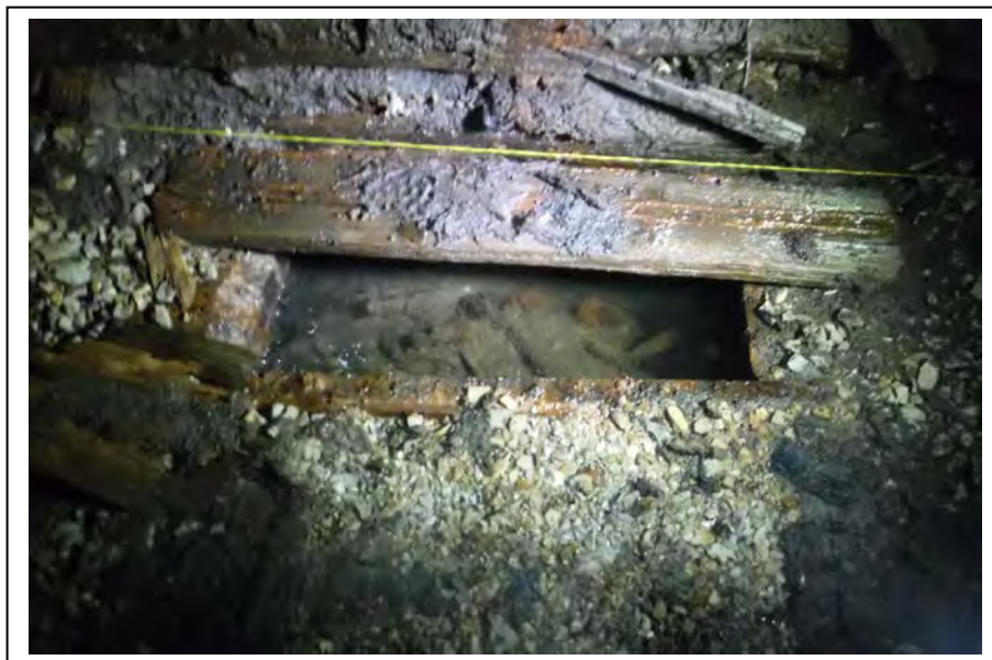
Photograph no 48: U/S sidewall at 100m Drainage running full but low flow
