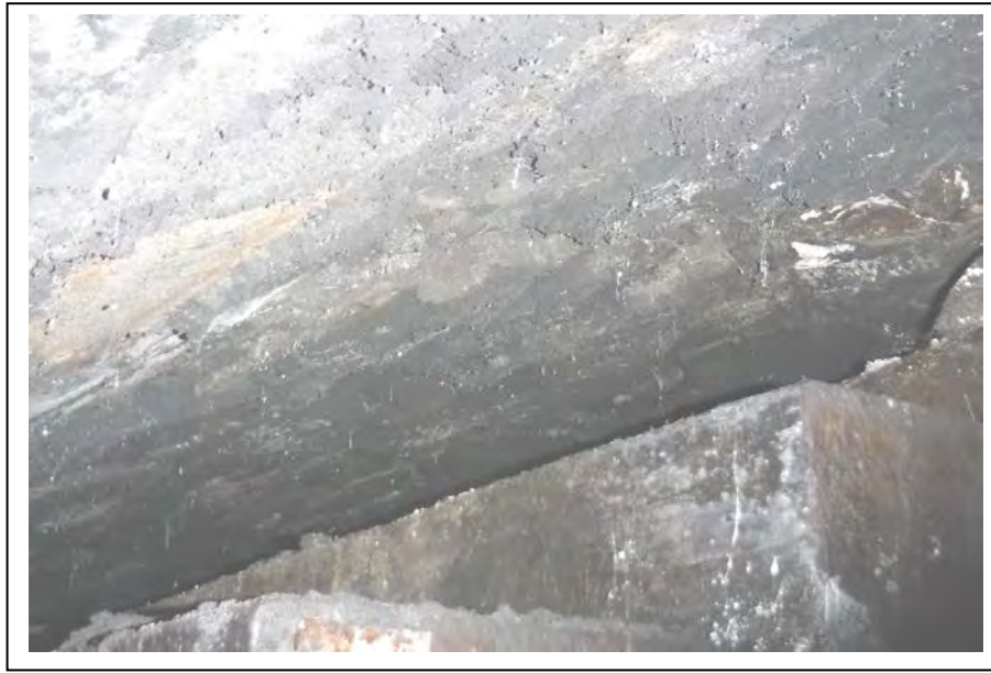
Photograph no C33: No evidence of packing to haunches of Cwg gap is typical of all elements, similar to crown
