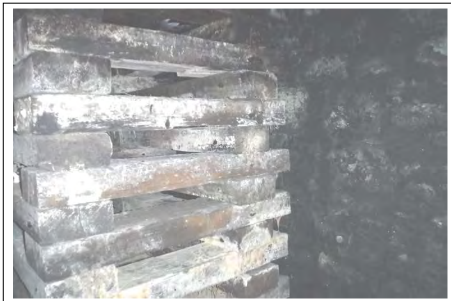
Photograph no C10: Cwg ② LE US sidewall
