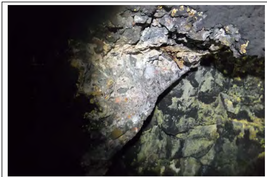
Photograph no 60: sidewall at 515m Large section of relieving arch CE face removed
