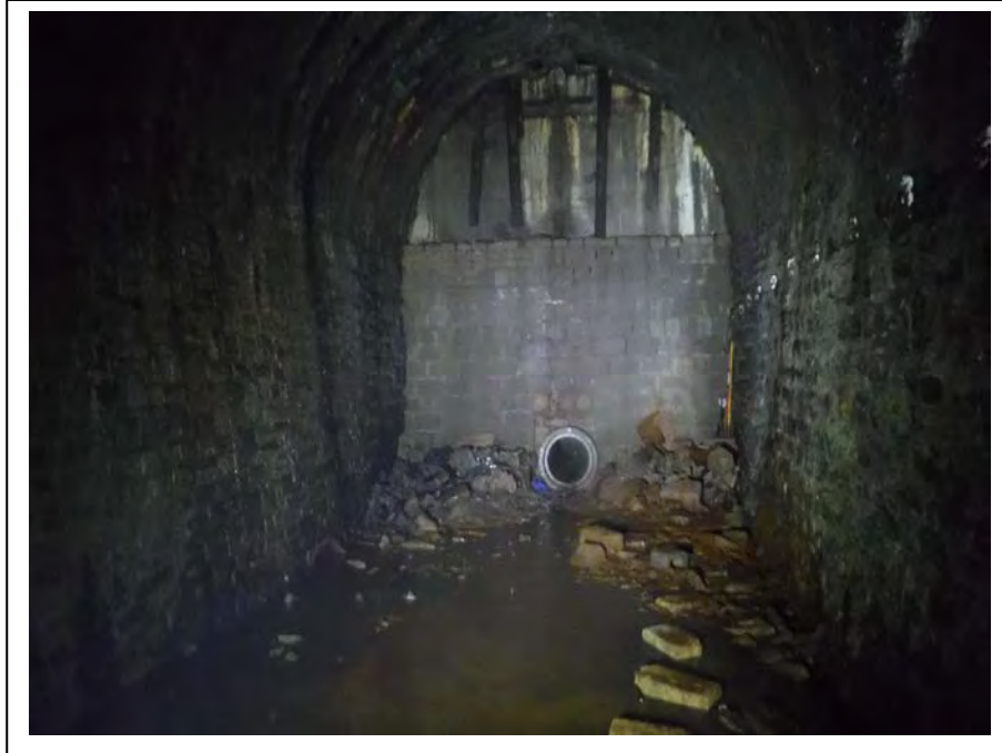
Photograph no 1: Diaphragm wall at 0m chainage (Blaencwm end)
