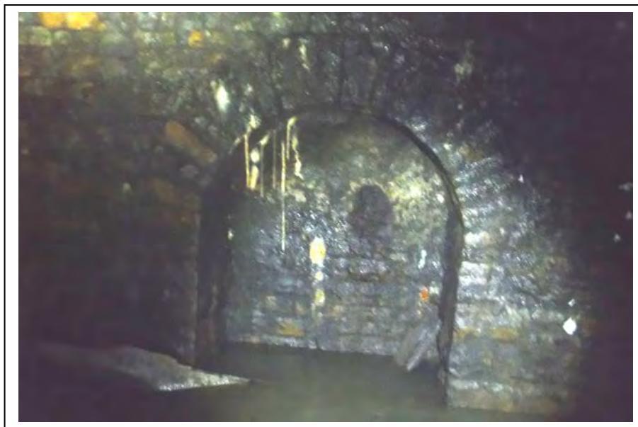
Photograph no 186: U/S refuge at 3050m
