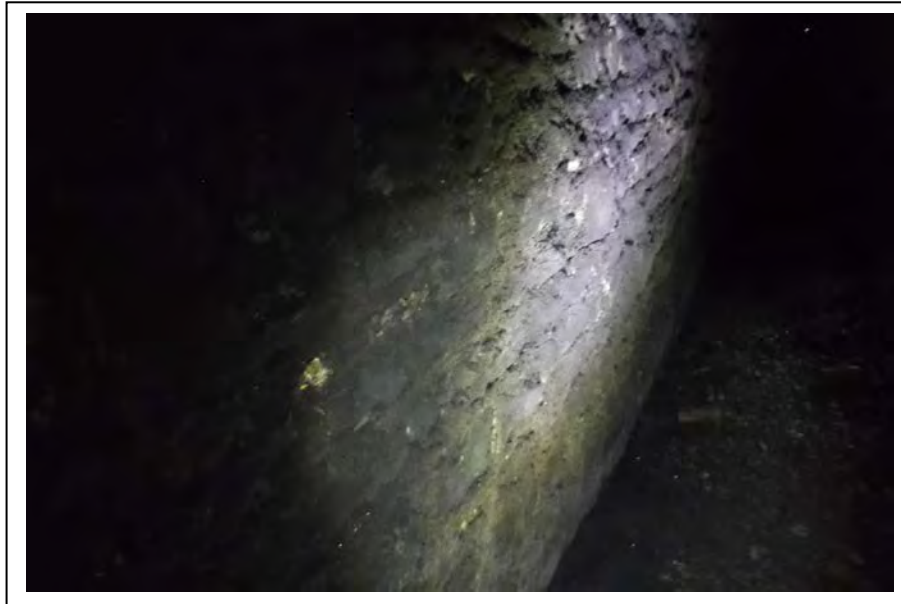
Photograph no 109: D/S haunch at 1020m Bulged area
