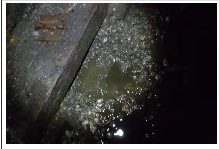
Photograph no 73: Bulk timber supports at base of ribs
