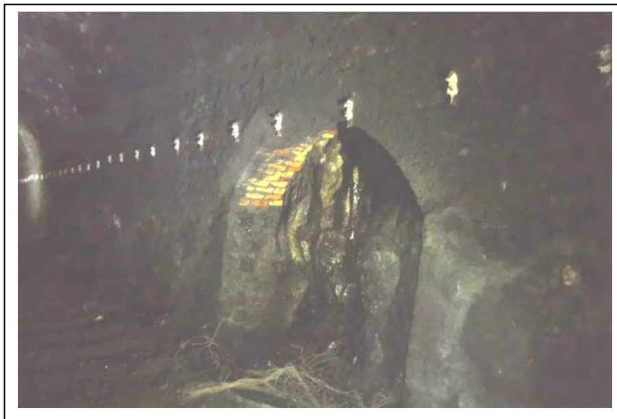
Photograph no 140: Typical views of relieving arches Taken at 2285m
