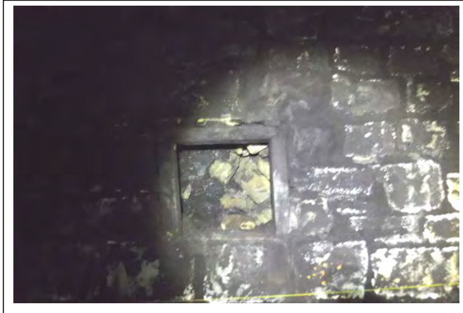
Photograph no 63: Sidewalls at 615m Deep recess (retrofit)
