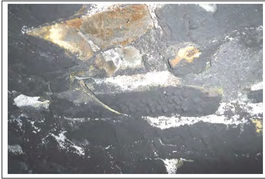
Photograph no C25: Fractured unit along hinge line at 1949m open 6mm
