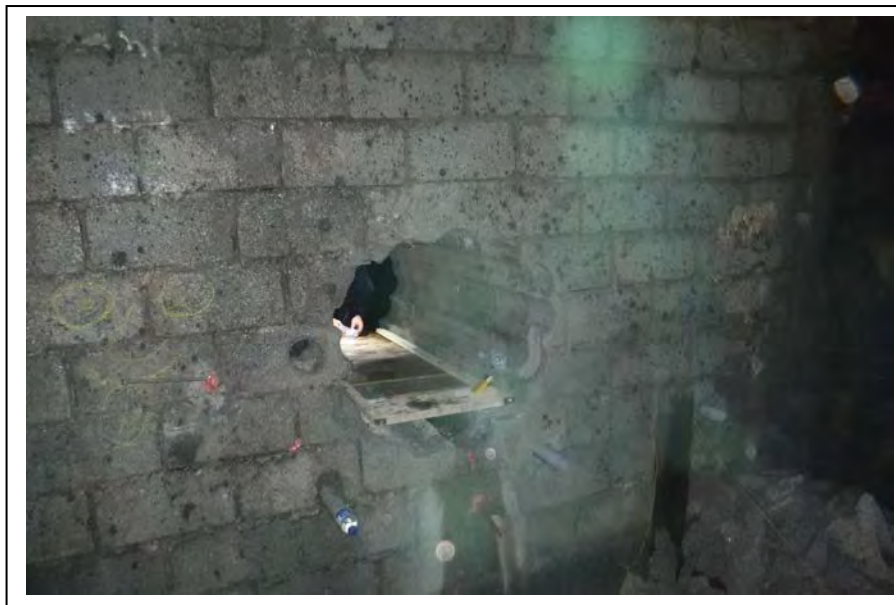
Photograph no 184: Crown at 3042m Newly cored access hole (May 2018)
