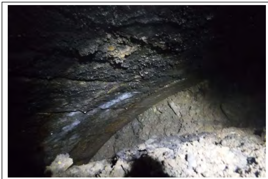
Photograph no 216: D/S haunch at 3132m Voussoirs in good condition
