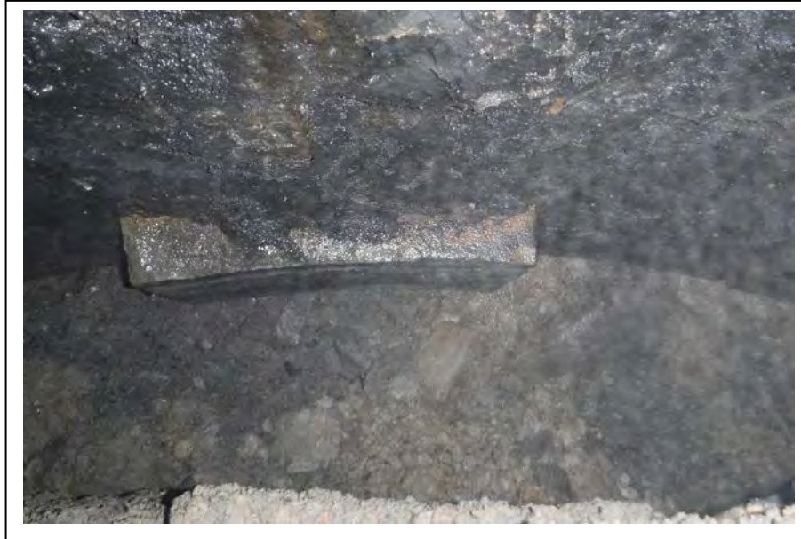
Photograph no 215: Crown at 3132m Tunnel keystone voussoir in good condition
