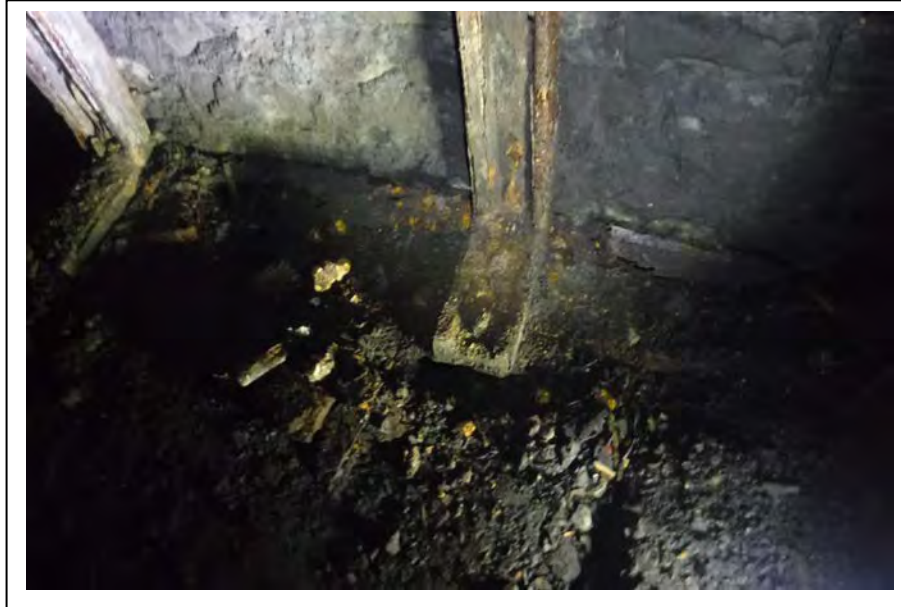
Photograph no 75: Cranked rib showing connection at base
