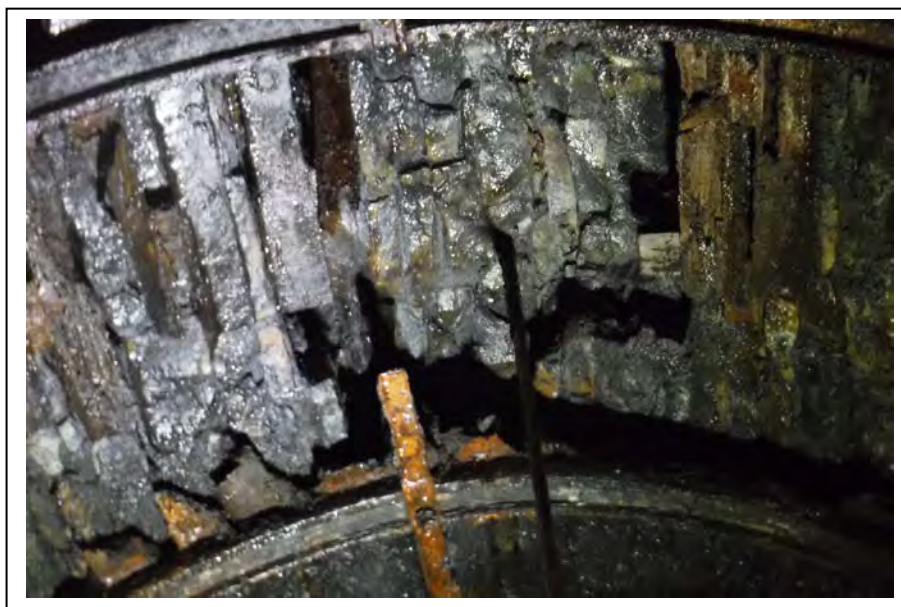
Photograph no 20: Crown at 97m (Ribs 20-21) Loss of section 1.1m wide x 300 deep max
