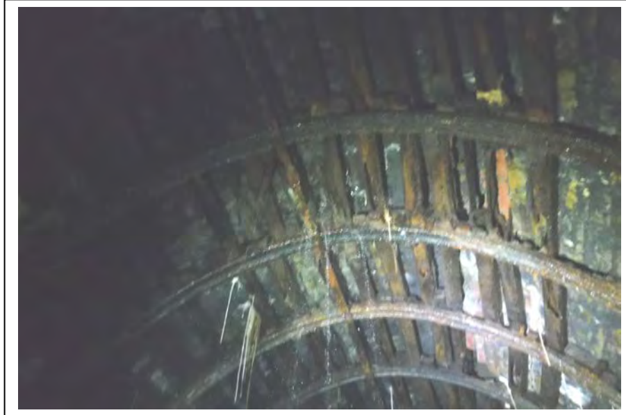
Photograph no 31: Crown at 146m Water running
