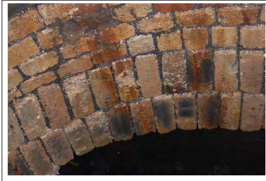
Photograph no 183: Base of shaft/ tunnel barrel
