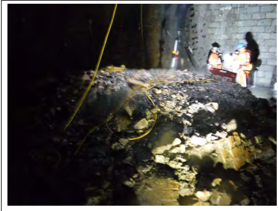
Photograph no 163: D/S haunch at 3034m Rubble to formation from imploded shaft "chimney"
