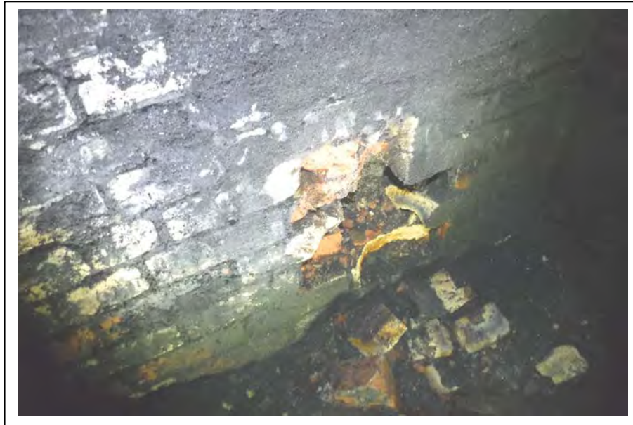
Photograph no 139: U/S refuge at 2140m Loss of section to rear of refuge 300 high x450 wide x 180 deep
