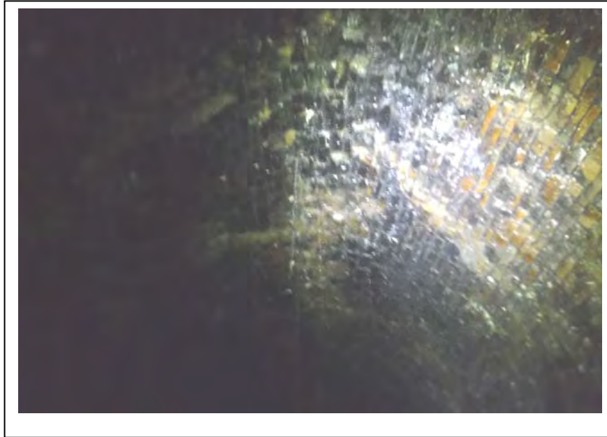
Photograph no 9: Crown at 45m Water running
