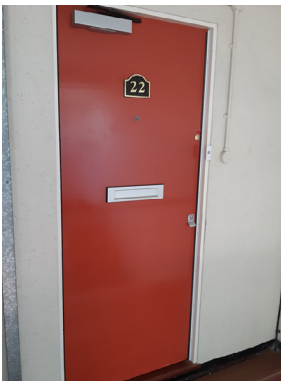
A typical timber flat entrance door
