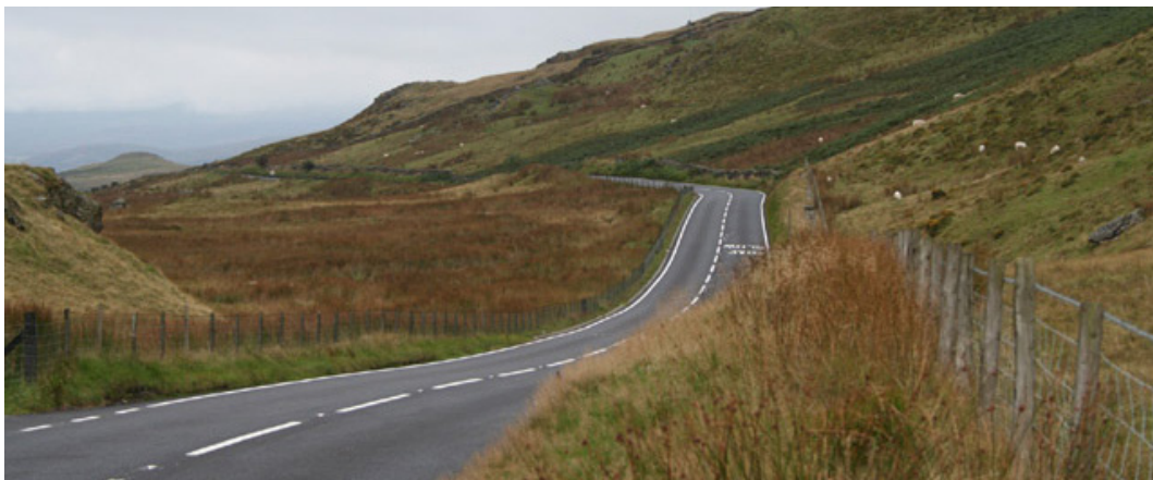
Fig.8 Example of rural section of the SRN A470 at Bwlch Oerddrws
