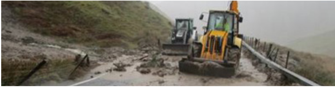
Fig.11 Risk Landslip Caused by heavy rainfall blocking the SRN
