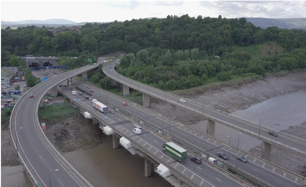
Fig.5 Maintenance of the M4 Usk Viaduct
