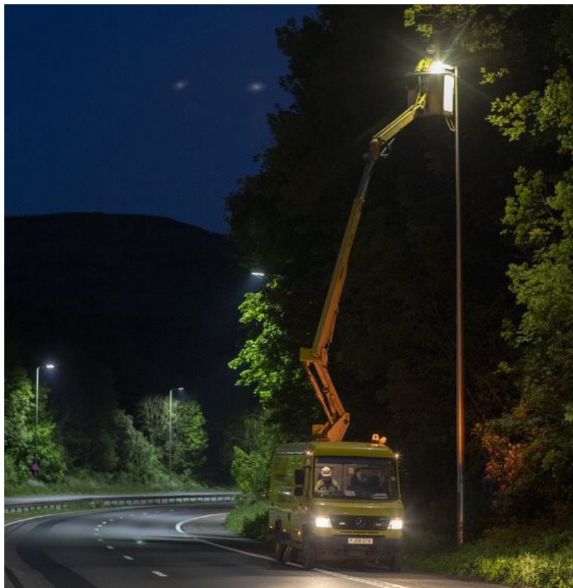
Fig.9 Example of Street Lighting Maintenance on the SRN
