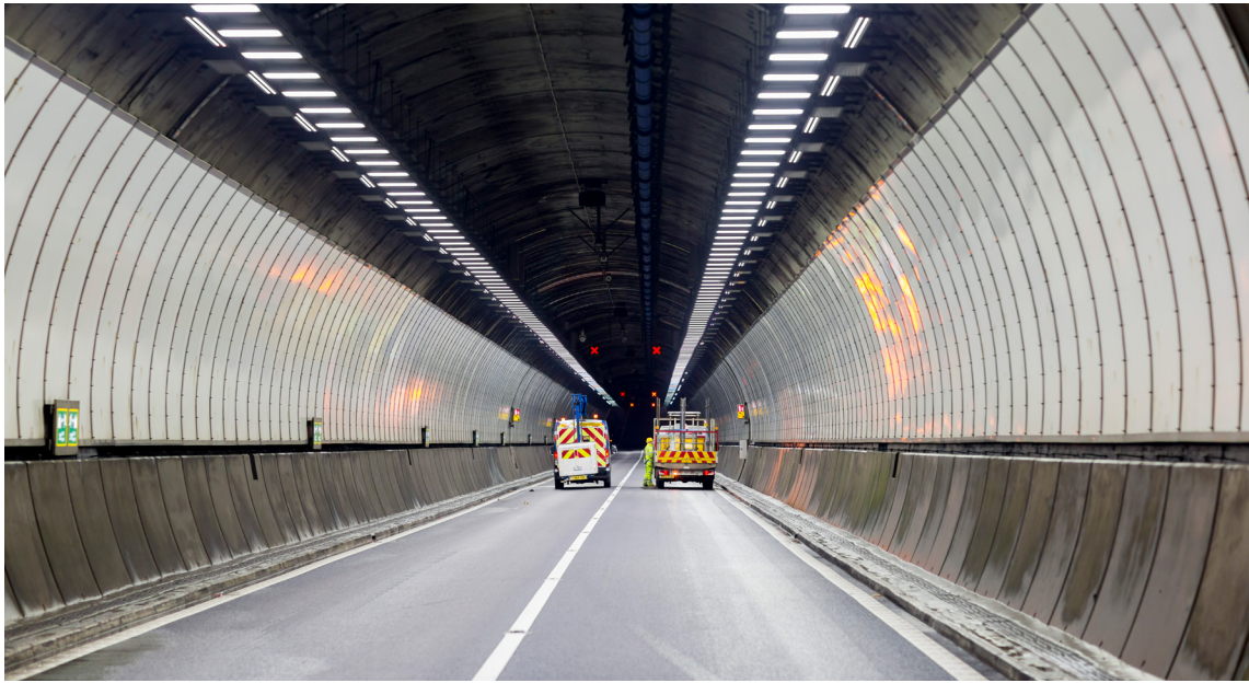
Fig.12 Undertaking maintenance in the M4 Brynglas Tunnel
