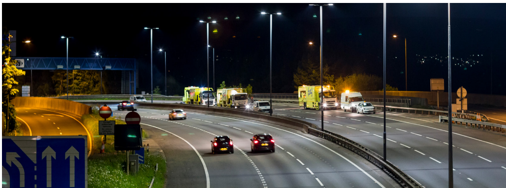
Fig.6 Lane closures for maintenance work M4 Malpas
