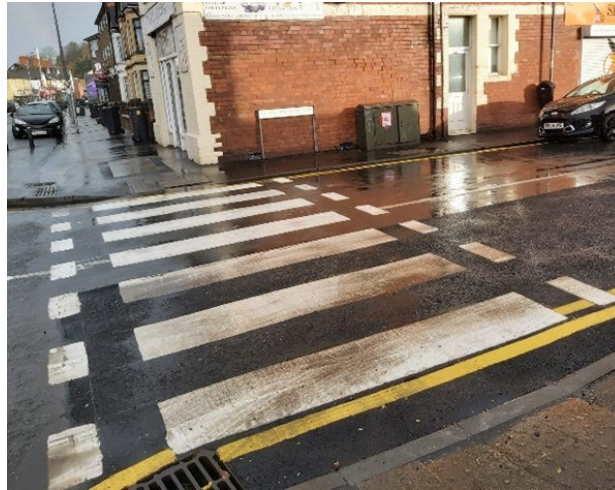
Figure 2: Example of the trial crossing at Location 2
