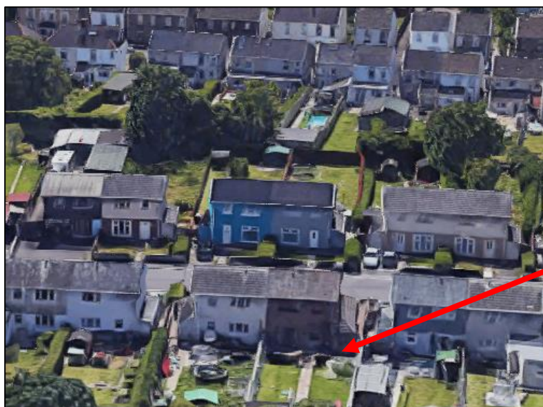
Figure 12: Example view of semi-detached properties, Swansea.
