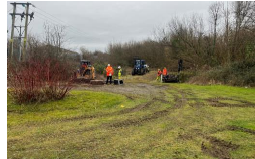
Ground survey works being carried out
