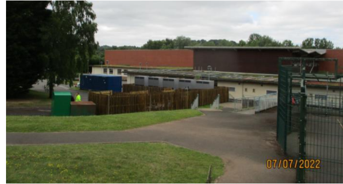
Integration of heat pumps into school site
