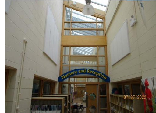
School corridor 'Integrated Solar PV'
