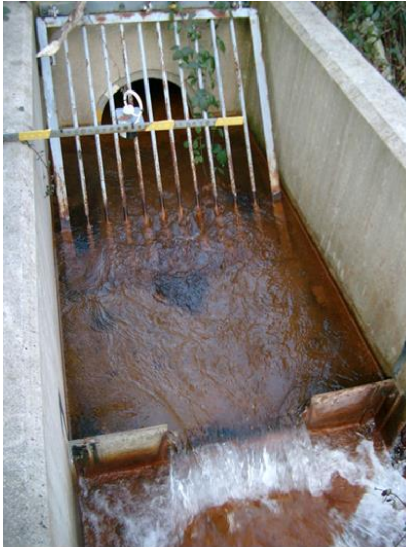
Figure 5.3: Photo of Plasdraw discharge
