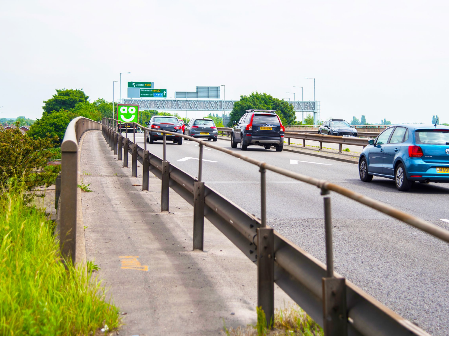
● Pont Afon Dyfrdwy’r A494 ar hyn o bryd (tua’r gogledd) ● Current A494 River Dee Bridge (northbound)
