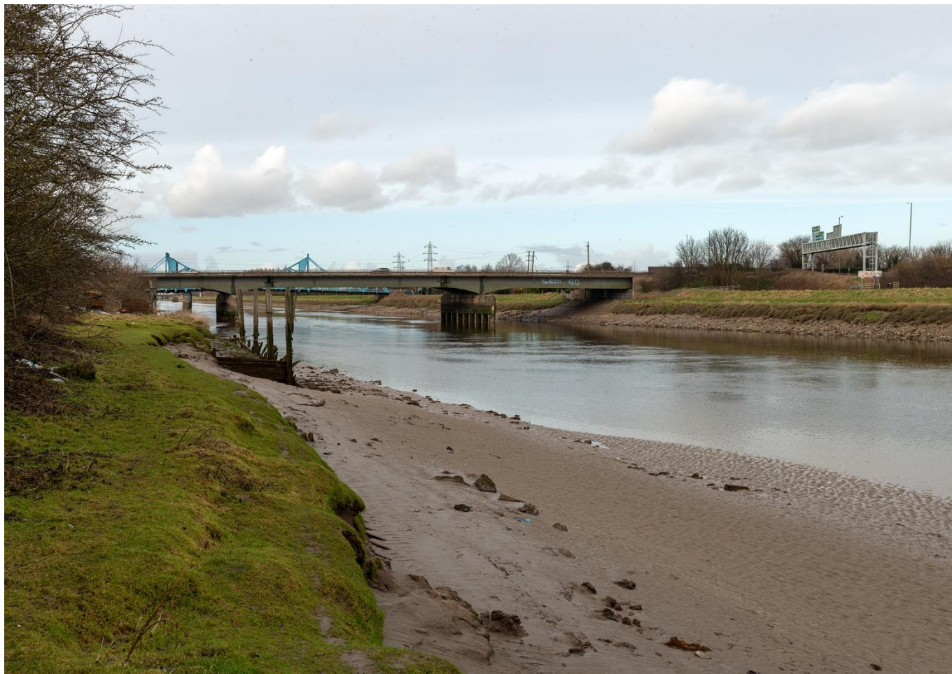
Figure 5: View downriver from River Dee embankment towards River Dee Bridge and A494 (Source: Richards, Moorehead & Laing)
