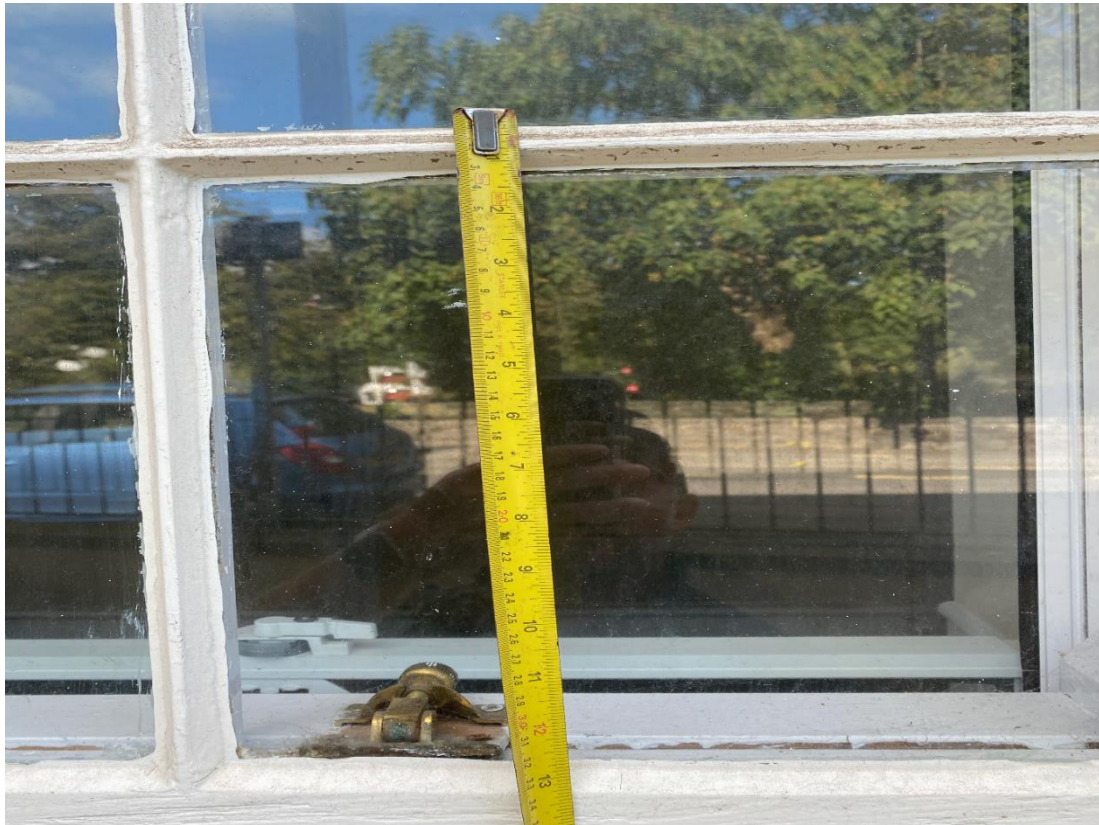
Figure 9 View to indicate size of pane of glass (Tape measure for scale)
