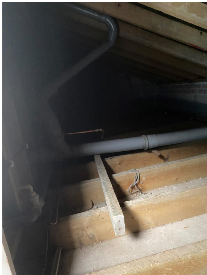
Figure 12 View of attic (Showing waste rainwater pipe)
