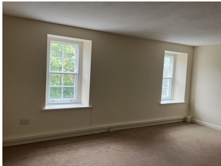
Figure 12 Evidence of deep window reveals
