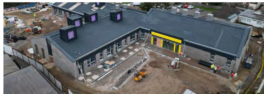
Llanilltud Primary School – drone view
