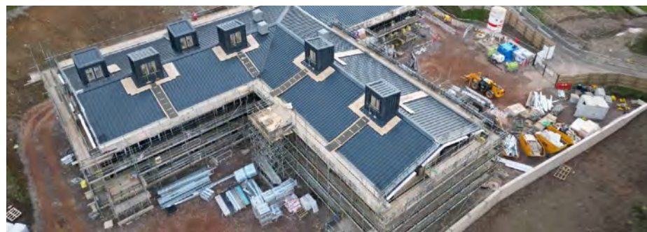
Penygawsi Primary School – drone view
