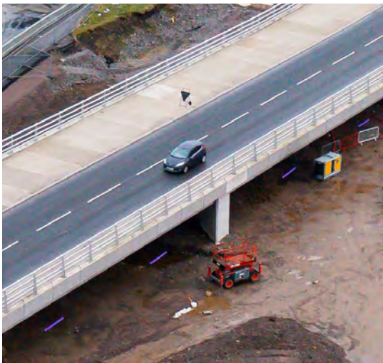
Trewaun West Bridge
