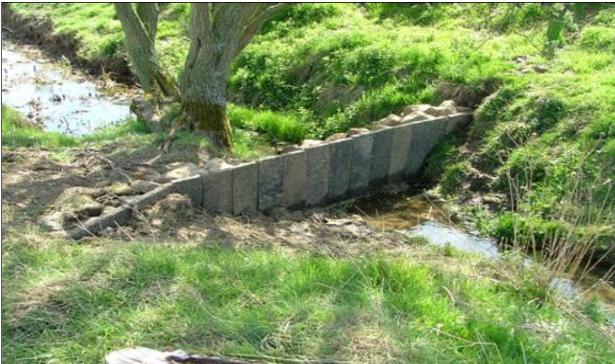
Seepage Barrier across a ditch.
