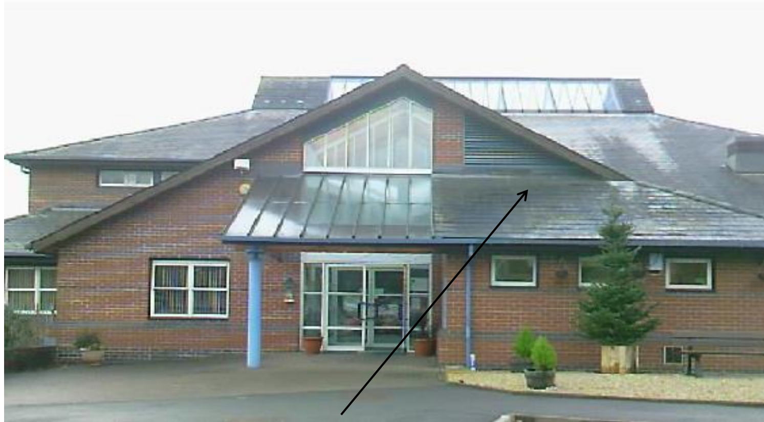
1990's Composite roof tiles – Asbestos Cement
