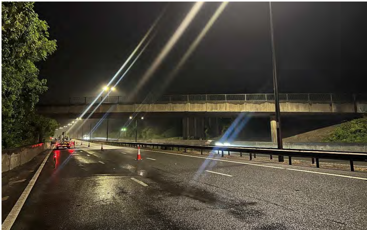
Photograph 2 - General view of the structure looking west.
