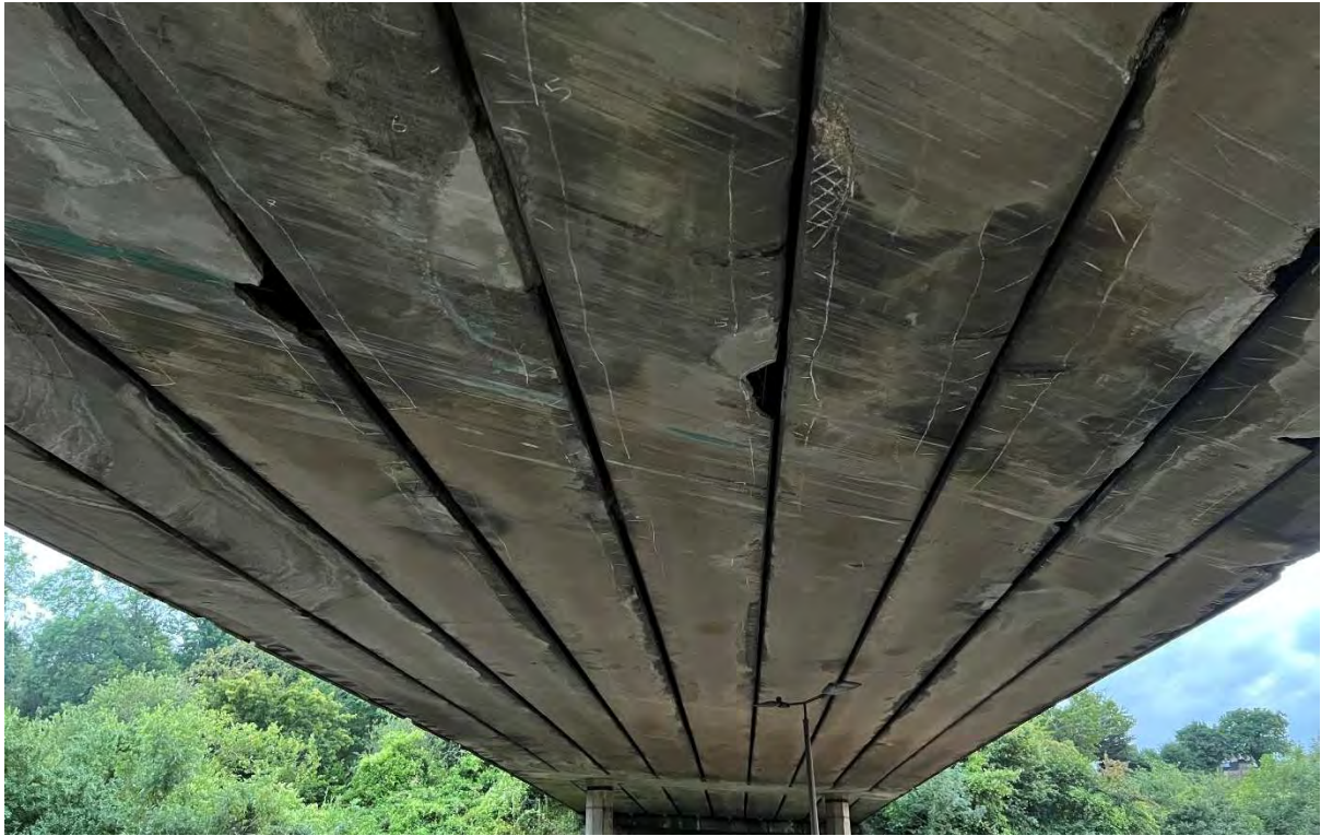
Photograph 5 - General view of the span 2 deck soffit looking south.
