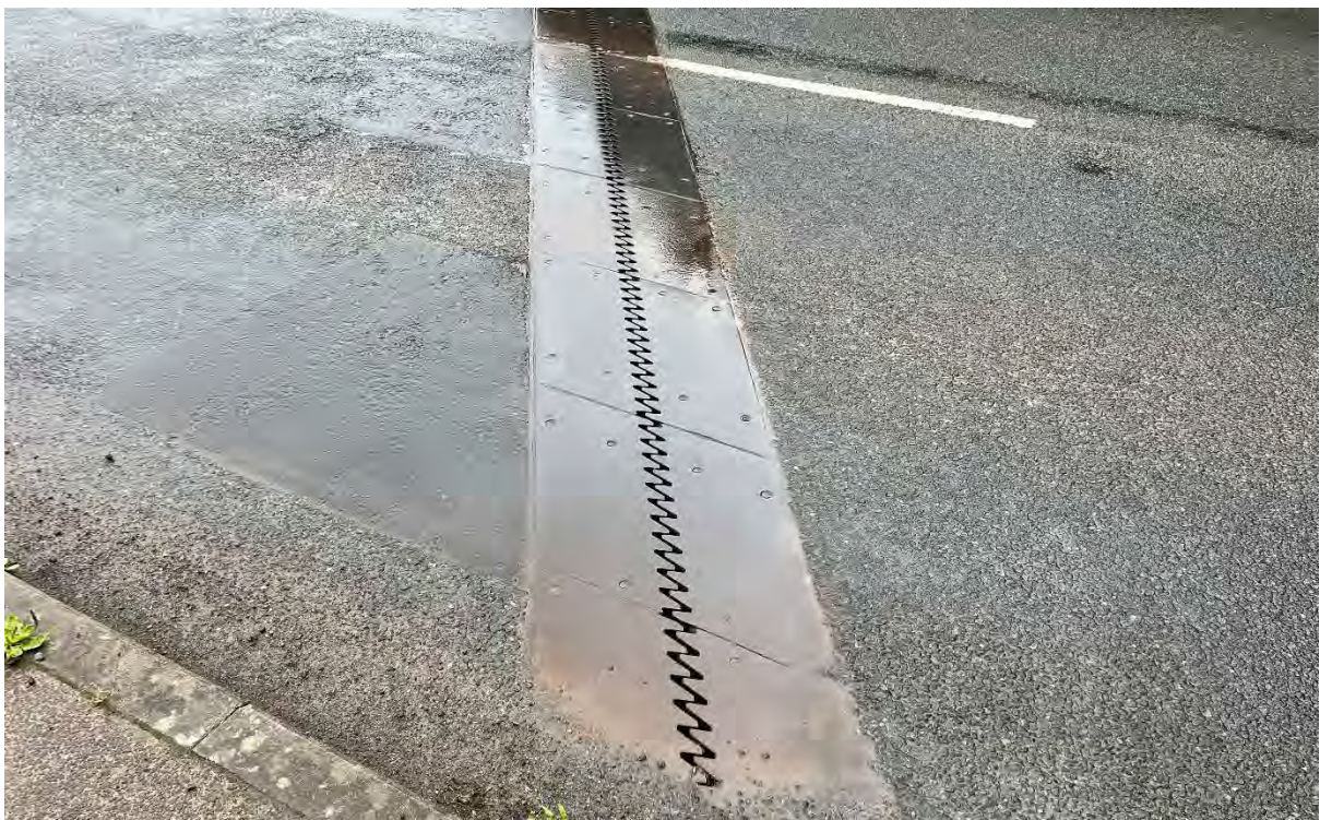
Photograph 72 - Span 1. South expansion joint.
