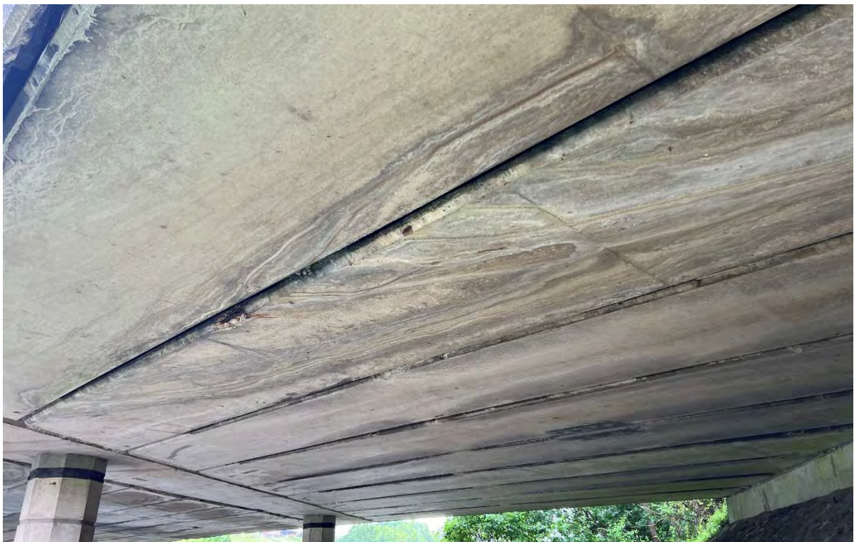
Photograph 6 - General view of the span 3 deck soffit looking east.
