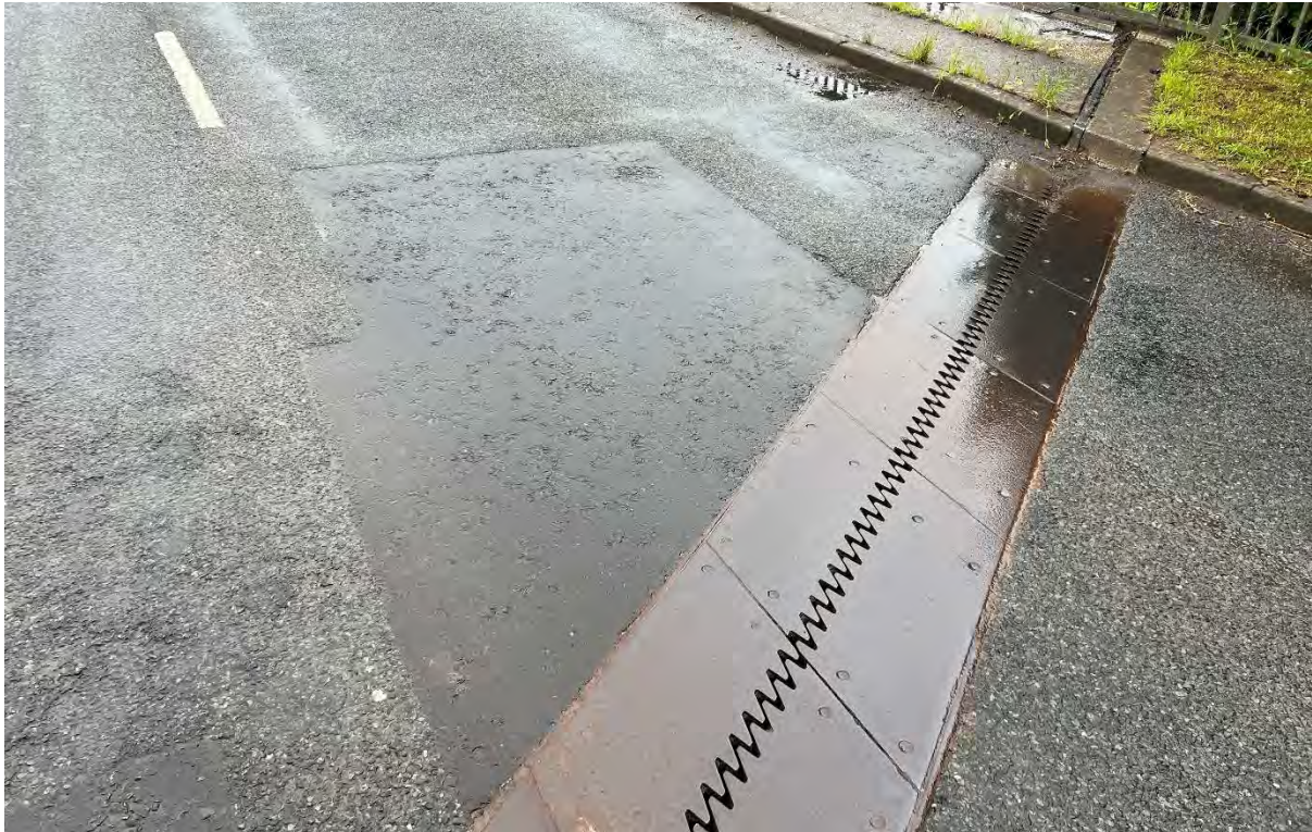
Photograph 81 - Span 2. Surfacing repair at north edge of southern expansion joint.
