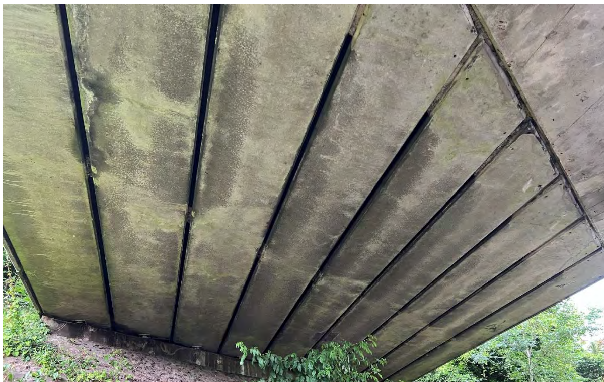
Photograph 4 - General view of the span 1 deck soffit looking south.
