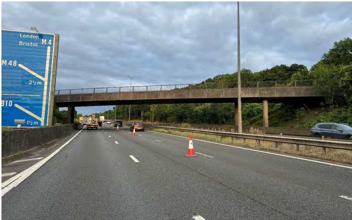
Photograph 1 - General view of the structure looking east.
